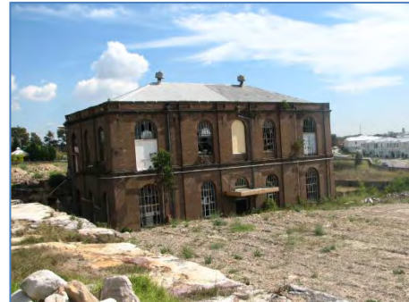
Photo 2: Former plumbers workshop
