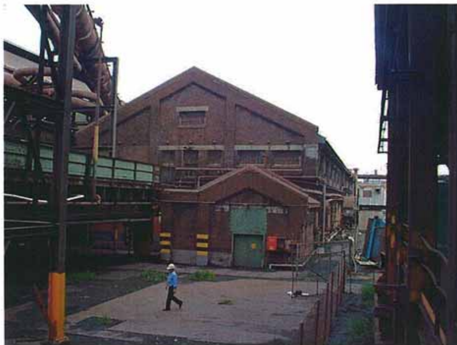
Figure 6.1 View West of Open Hearth Change House's Eastern facade. Shows Main 2 storey building with late single storey extension in foreground for tar fuel pump house.
