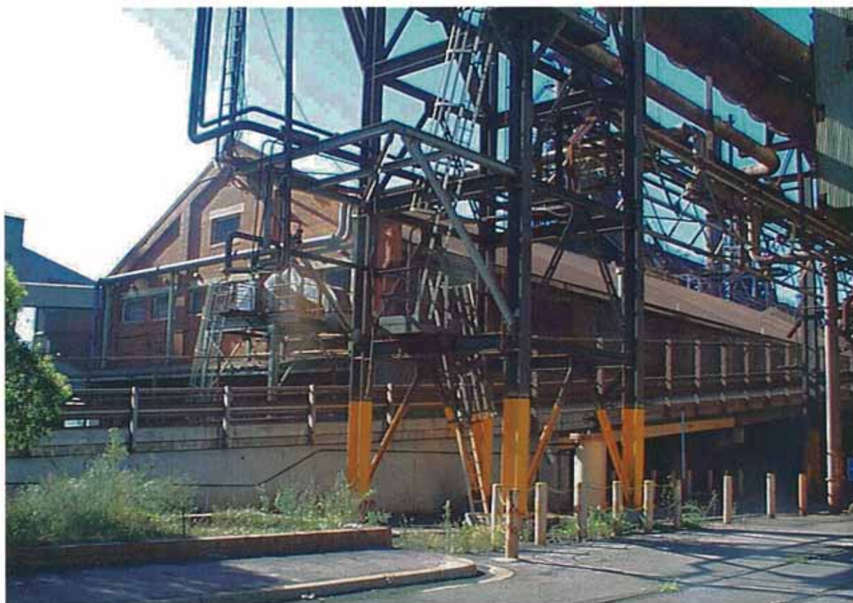
Figure 0.1 View North – East of Open Hearth Bath House showing West and South facades overlaid with the later added B.O.S. scrap feed ramp and pipe-work framing.
