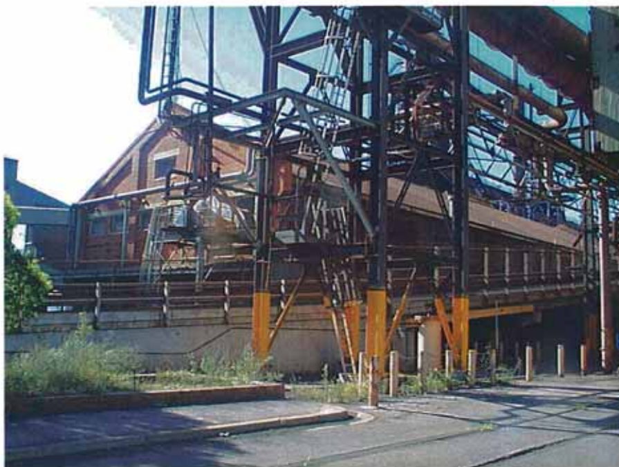
Figure 6.3 View North – East of Open Hearth Bath House showing West and South facades overlaid with the later added B.O.S. scrap feed ramp and pipe-work framing.
