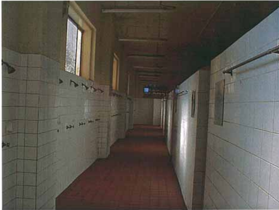
Figure 6.10 View East along North side of showers to Open Hearth Bath House. Showers have been heavily modified to run East – West. Showers originally ran North – South with division wall at each. Wall panel at centre / external wall pier.
