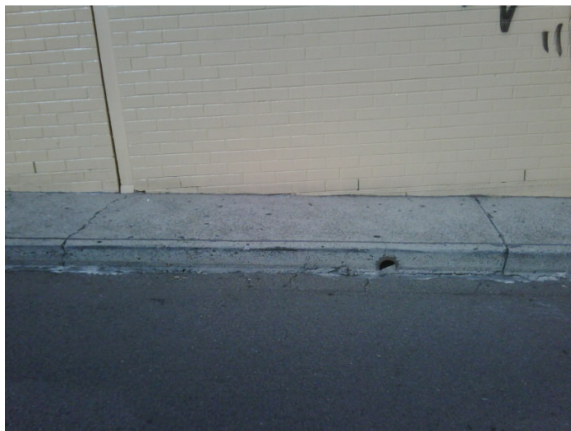
Photo 6: Kerb connection in Christie Lane (Connection 5)
