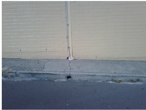
Photo 5: Kerb connection in Christie Lane (Connection 4)
