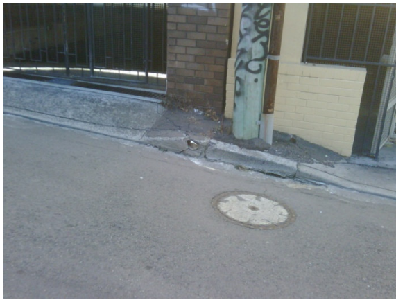
Photo 4: Kerb connection in Christie Lane (Connection 3)
