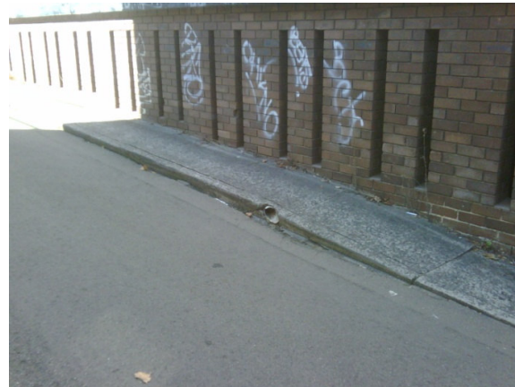
Photo 3: Kerb connection in Christie Lane (Connection 2)
