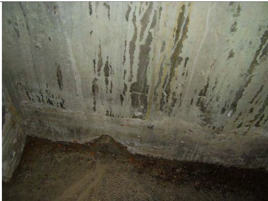
Figure 3: Observed groundwater seepage at the bottom of a retaining wall
