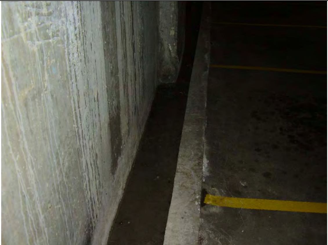
Figure 2: Observed groundwater seepage at the bottom of a retaining wall
