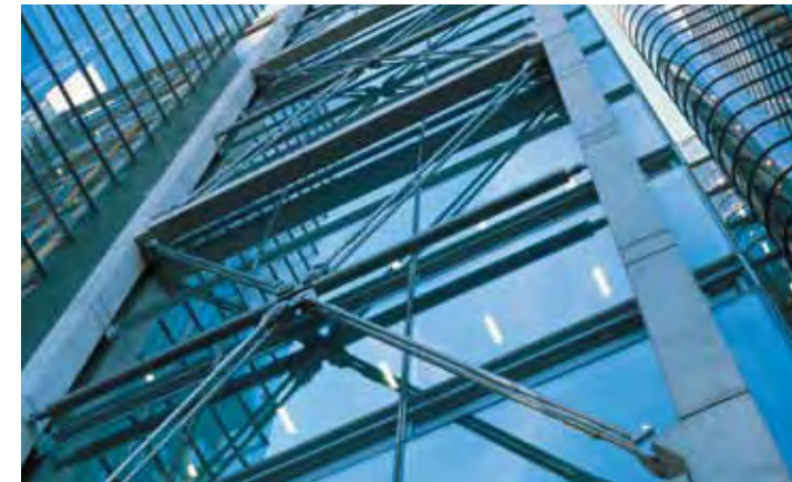
An expressed structural frame - 88 Wood Street, London
