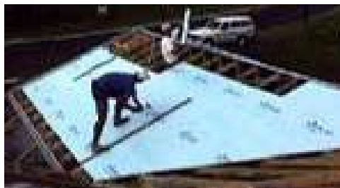
Figure 4 Installation of Styrofoam Insulation System
