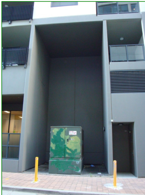
Figure 3: Alcove Installed Kiosk Transformer (Not a Standard Design)
