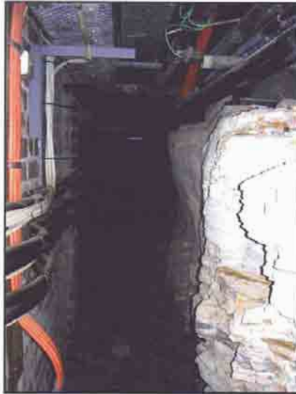
Photo 1: Basement wall to the left and shale bedrock exposure to the right
