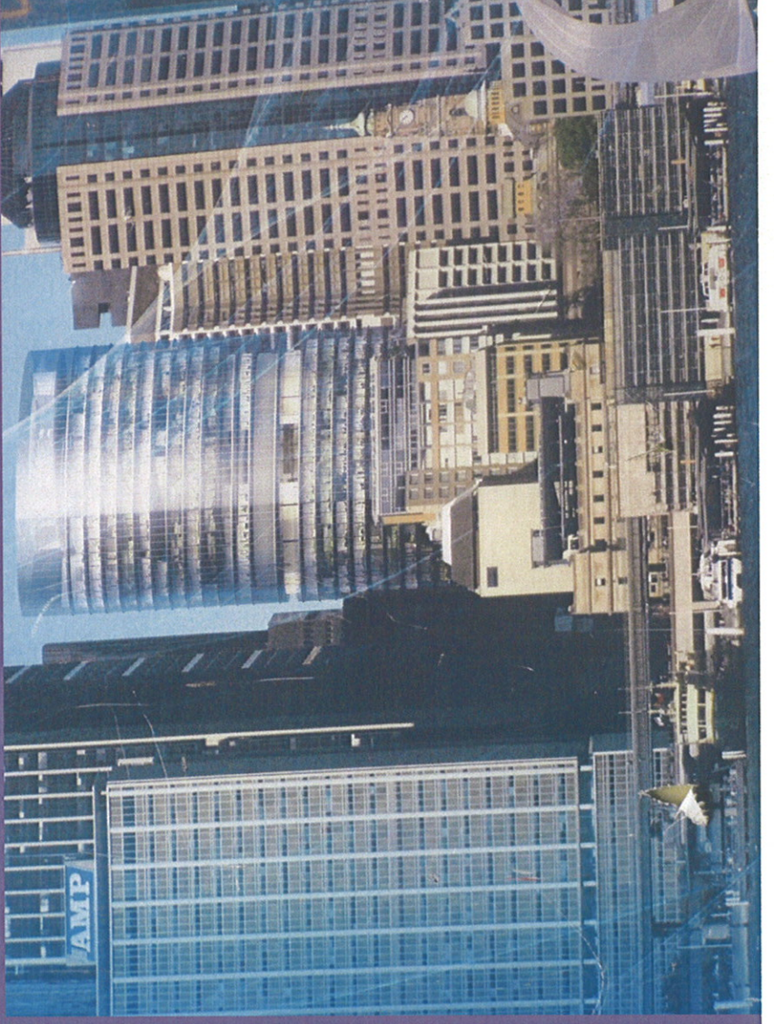
1 Bligh Street = new sustainable design = curved shape + twin outer walls + atrium inside.
