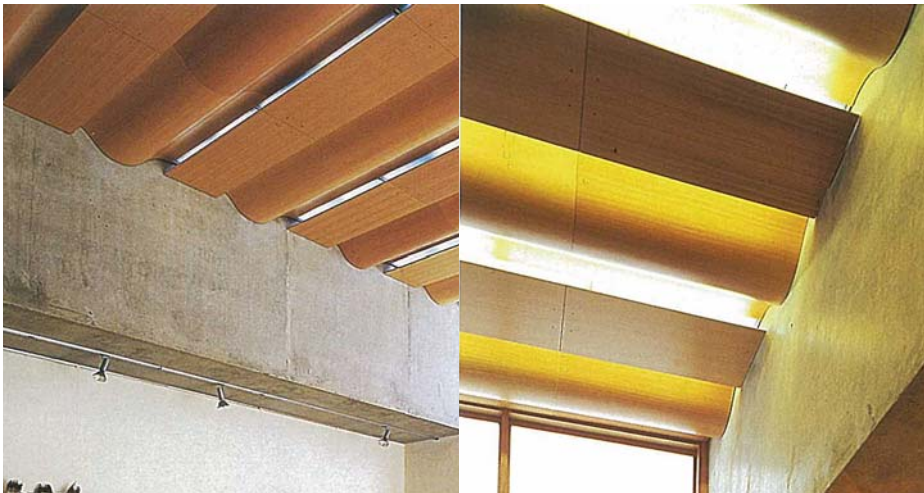
Fig. 26 // Roof forms that allows natural lighting into internal spaces
