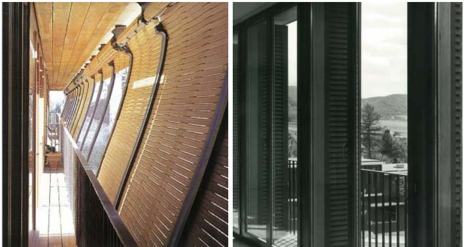
Fig. 24 // Balconies with operable shading devices to control solar access
