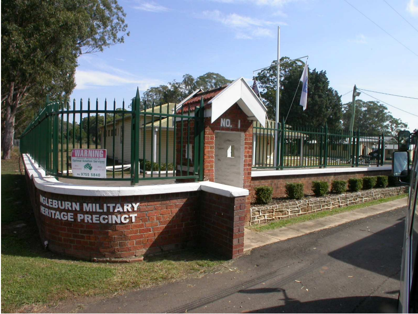
Figure 8c - View of the Ingleburn Military Heritage Precinct from Campbelltown Road
