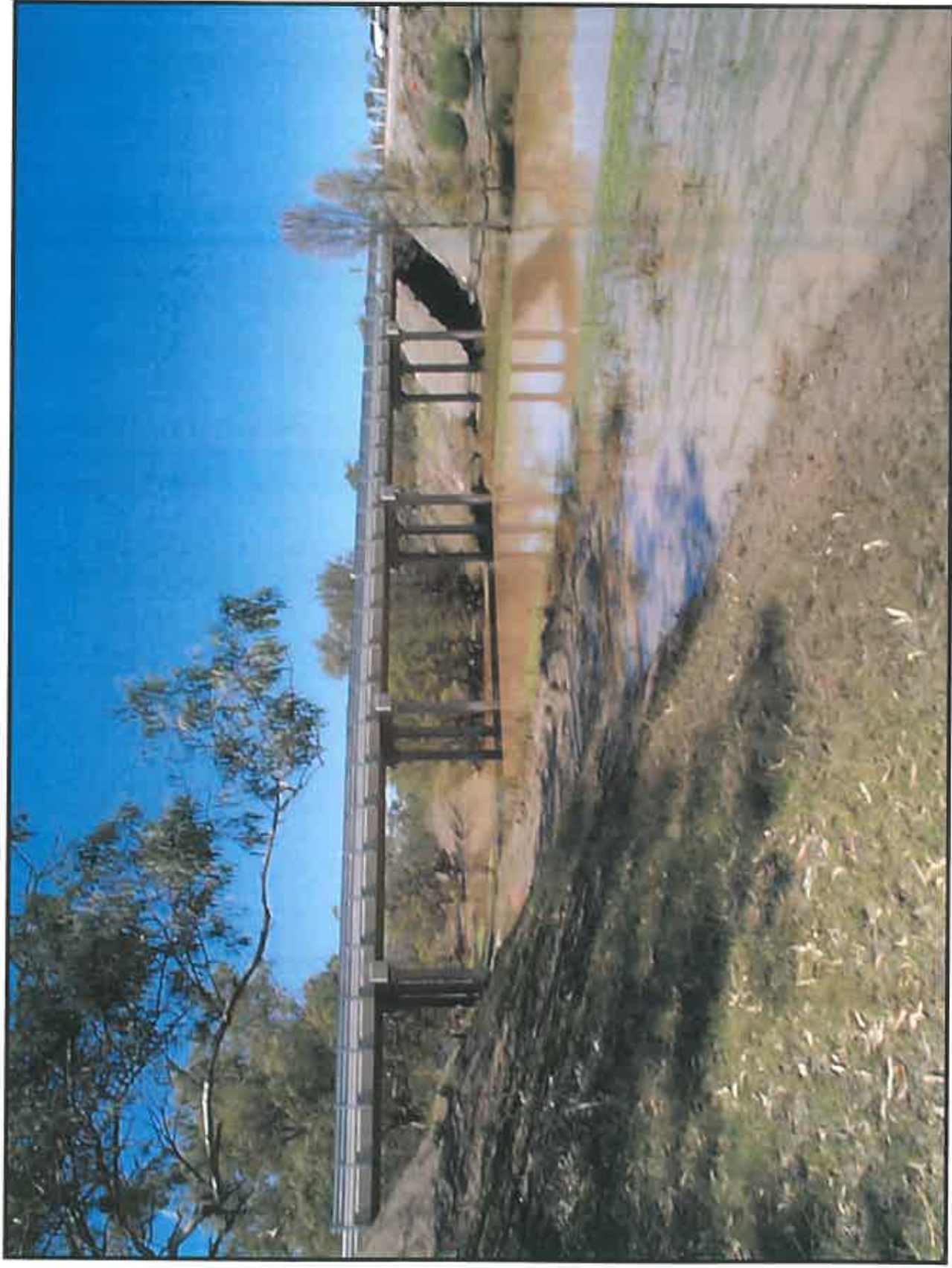
Completed 5 span (5 x 12m) M-LOCK ® Bridge over the Culgoa River - Goodooga, NSW.
