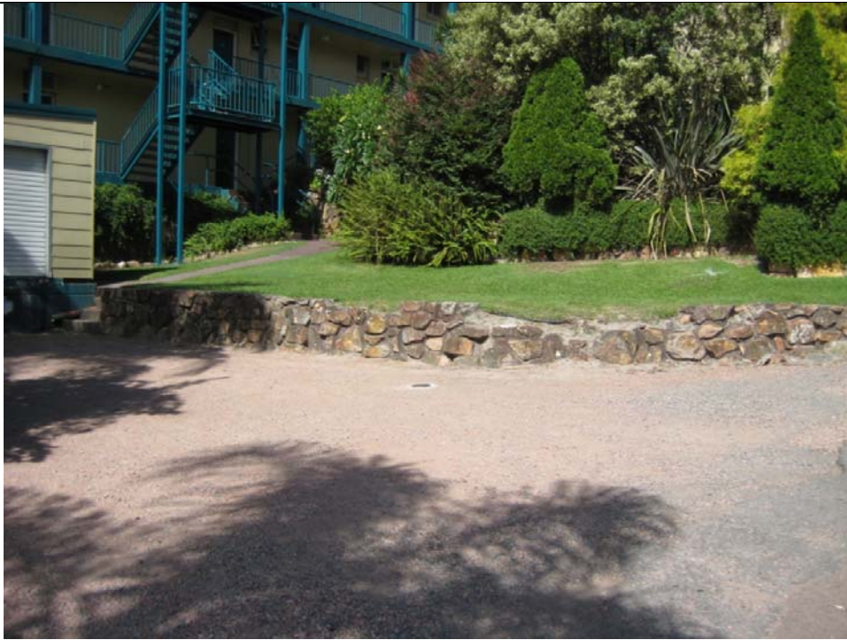
Photograph 3: Looking near the central portion of the main accommodation area of the hotel. Note the groundwater monitoring well (the circular object in front of the stone wall); one of two monitoring wells at the site.
