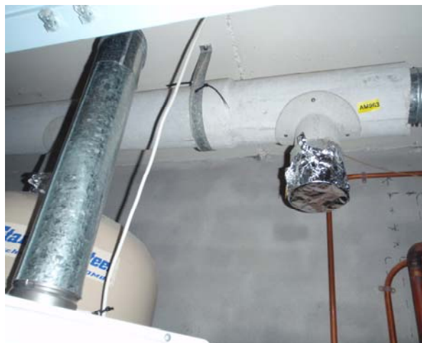
Photograph 5: Asbestos cement debris - Internal: boiler cupboard within bathroom.
