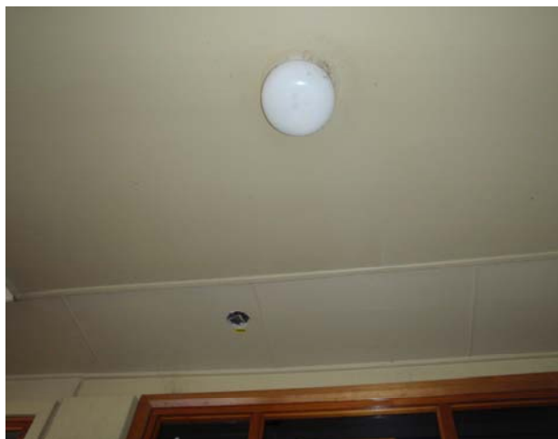
Photograph 4: Formed asbestos cement caps on flue - Internal: boiler cupboard within bathroom.
