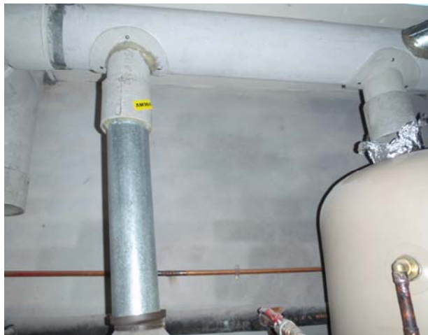
Photograph 4: Formed asbestos cement caps on flue - Internal: boiler cupboard within bathroom.
