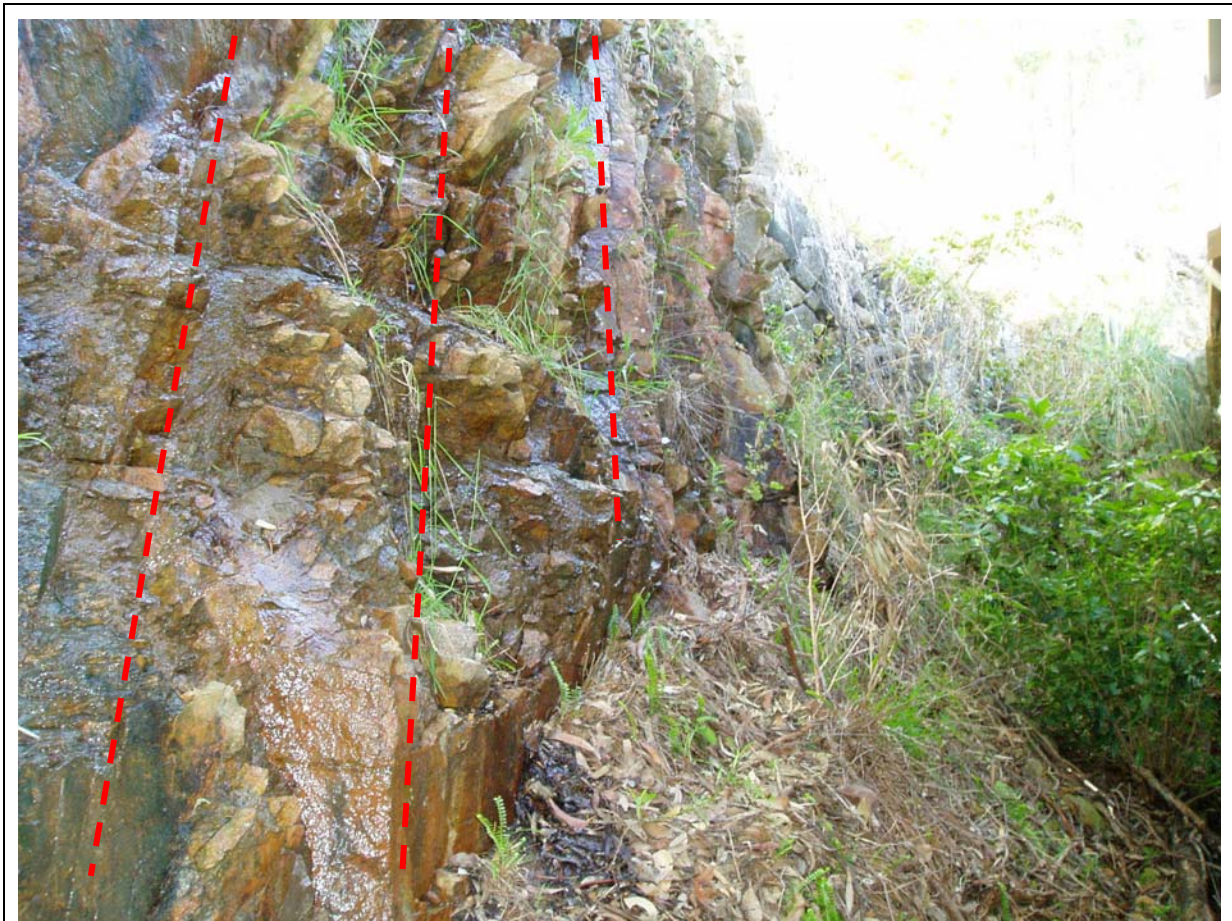
Photograph 1 – Cutting behind the Sailing and Aquatic Club to the east of the site, red dashed line annotates the predominant columnar structure of the rhyodacite rock.
