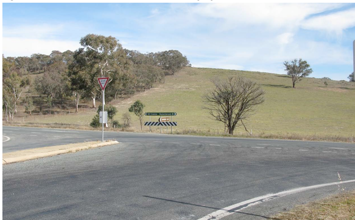
Figure 13.1 Intersection at Old Cooma Road and Googong Dam Road
