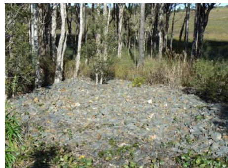
Plate 14: Broken rock to eliminate scour used by Council along Ocean Drive may prove suitable for stormwater discharge outlet into Duchess Creek
