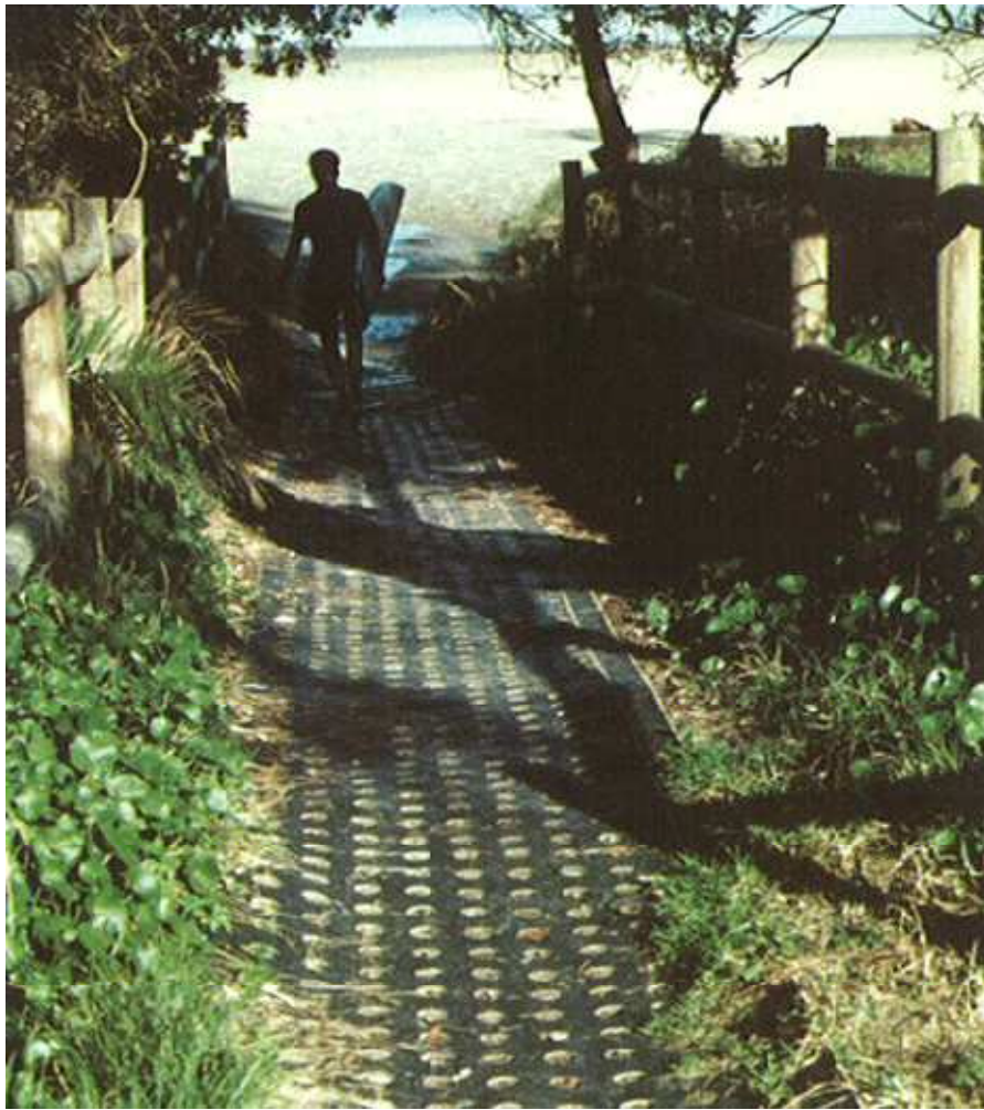
Figure 5.3 –Conveyor belt pathway (Coastal Dune Management , NSW Government, 2001)
