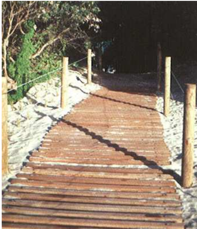
Figure 5.1 – Board and chain accessway (Coastal Dune Management, NSW Government, 2001)
