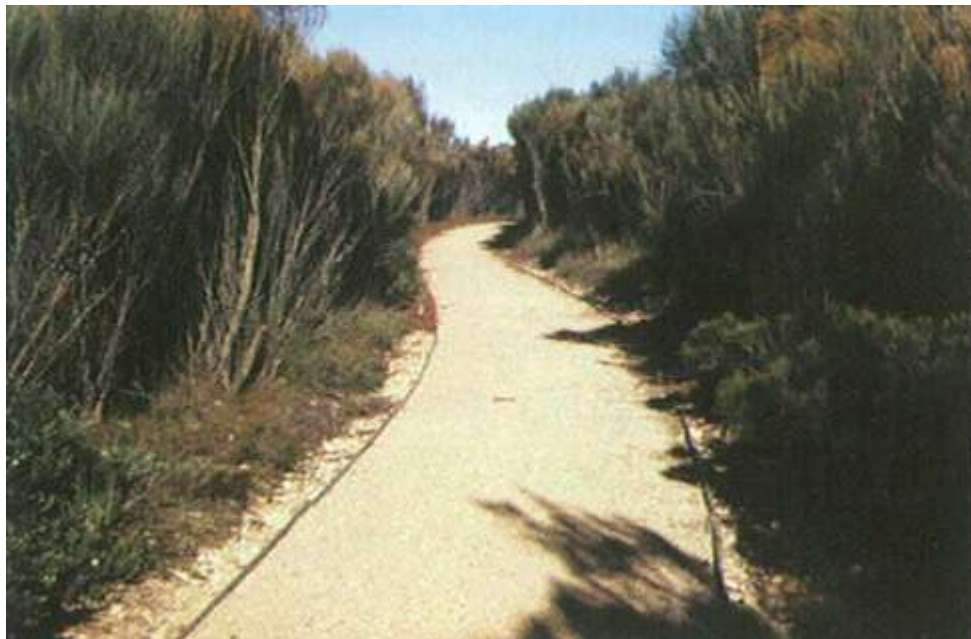
Figure 5.2 – Crushed sandstone accessway (Coastal Dune Management, NSW Government, 2001)
