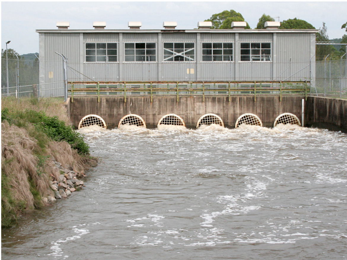
Photograph No 4: Balickera Pumps looking upstream to the pump station outlet. When this photo was taken, six pumps were in operation and the installed pump capacity was around 1350ML/day. (The 2004 licence indicates that the approved capacity was 1400ML/d). Note that recently two additional pumps were installed taking the installed capacity of the pump station to approximately 1800ML/day although actual pumping rates are dependent on levels in Grahamstown Dam and may vary. HWC's hydrologic model, SoMo, which has been utilised in the EAR and the EASR, has assumed a pump capacity of 1650ML/day. This would appear a reasonable assumption and provides for some 'downtime' when pumps may not be fully operational. NOW have advised that HWC's existing licence allows them to extract 1810ML/d and there is provision for them to increase this to 2000ML/d in the future.
