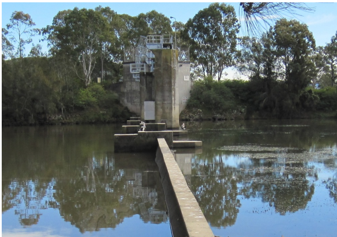
Photograph No 3: Seaham Weir provides a barrier across the Lower Williams Estuary and was constructed around 1967-1970. Vertical lift gates allow catchment flows that have collected on the upstream side of the structure to be released in pulses, typically of 1-1.5 hour duration. This maintains the upstream weir levels within the normal operating range. During flood times, the gates are lifted clear of the weir pool level until such time as the weir pool has dropped back to the normal operating range. Although not shown in the photograph, there is also a small fishway constructed through the weir which HWC have estimated passes approximately 5ML/d on average over a normal 28 day tidal cycle. This fishway is proposed to be upgraded to improve fish passage and allow up to 20ML/d to pass the weir. Note that in very dry times, the upstream water level can drop below the downstream level (due to evaporation and other losses) and both the existing and proposed fishway flow 'backwards'.
