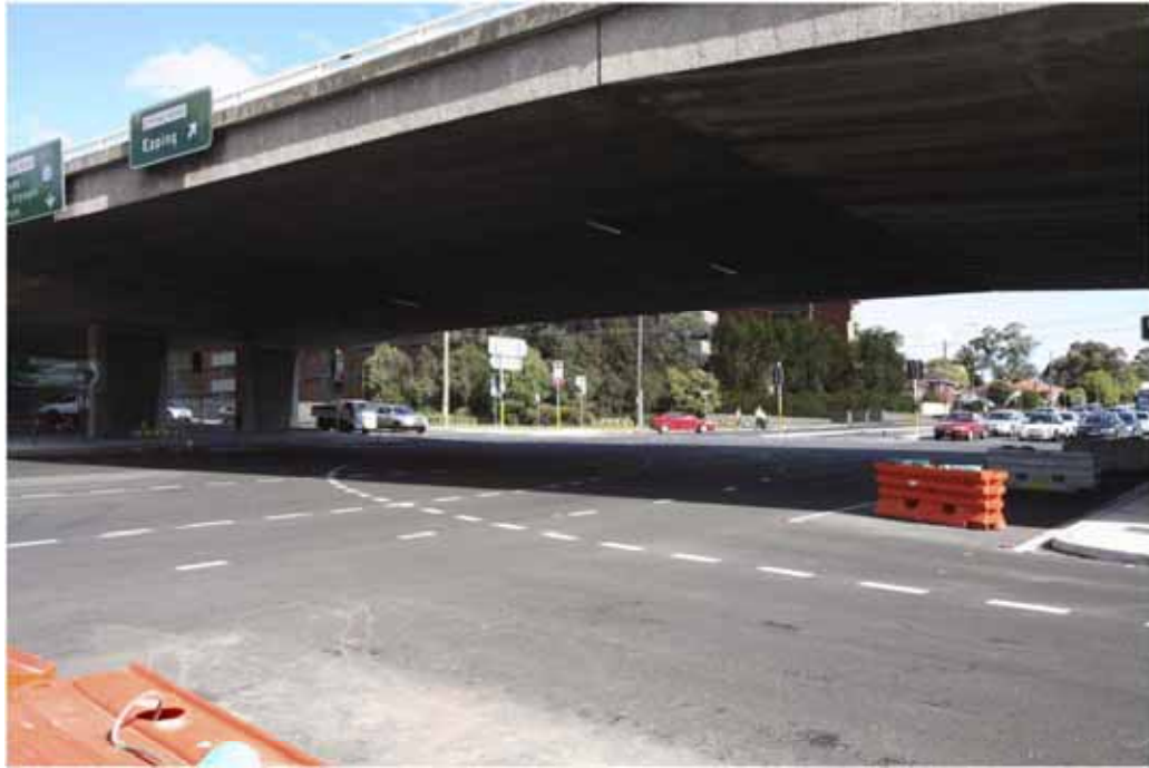
01 VIEW 1 - LOOKING SOUTH FROM EPPING ROAD OVERPASS
