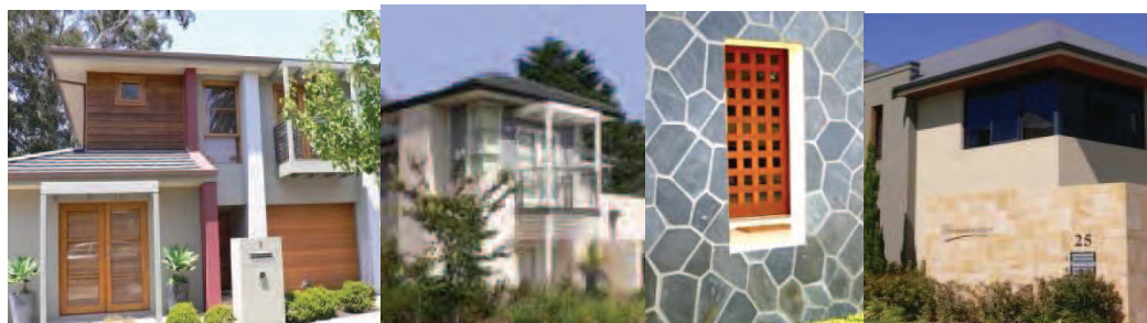
Figure 3.1.3.3 Desirable primary road façade design features - timber, stone, wide eaves, porches and verandas
