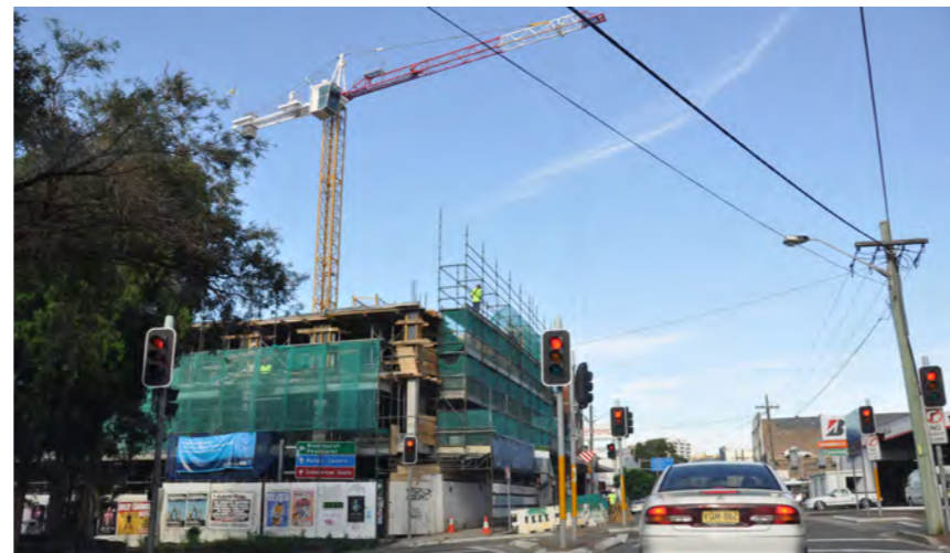
14 8 STOREY RESIDENTIAL (UNDER CONSTRUCTION)_9-13 TREACY ST
