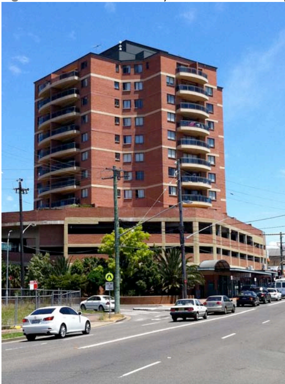
Figure 5 – View of 12 storey mixed use development
