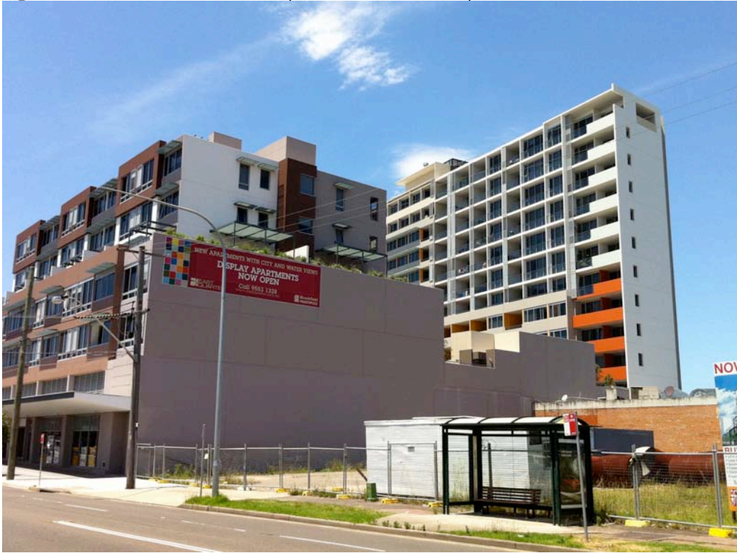
Figure 4 – View of East Quarter (former AMCOR site)
