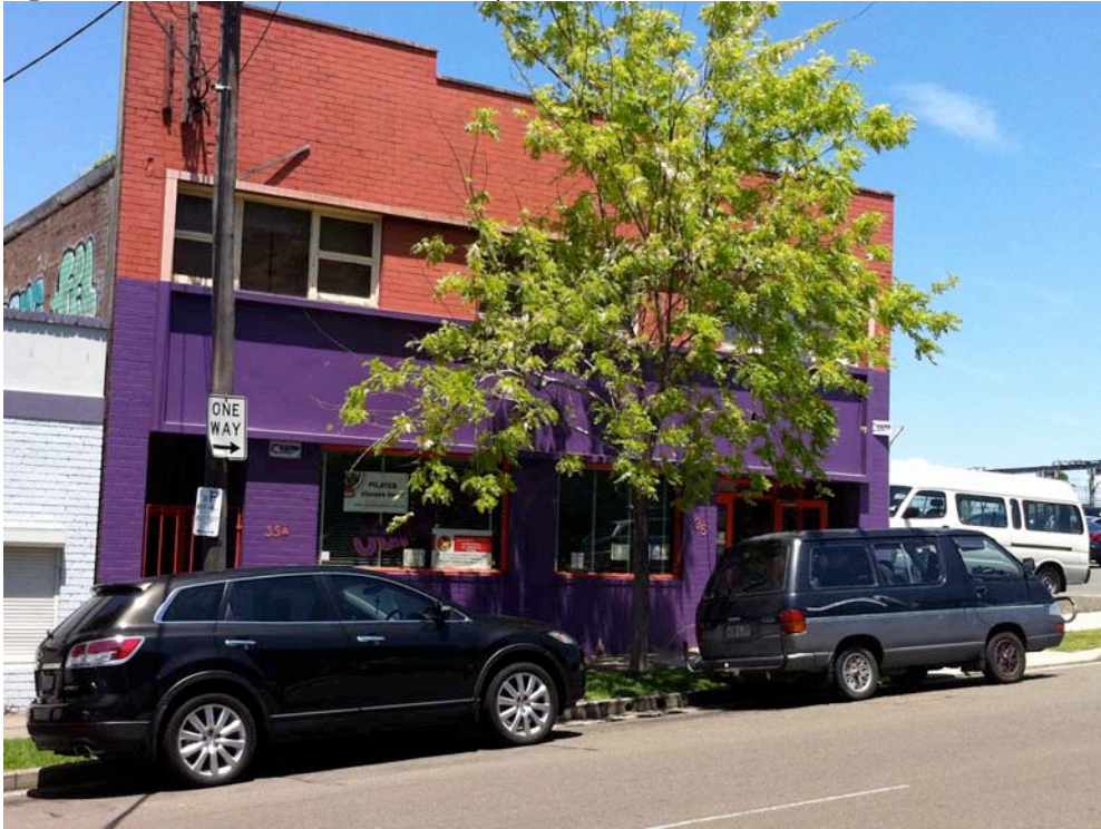
Figure 13 - View of 35 & 35A Treacy Street
