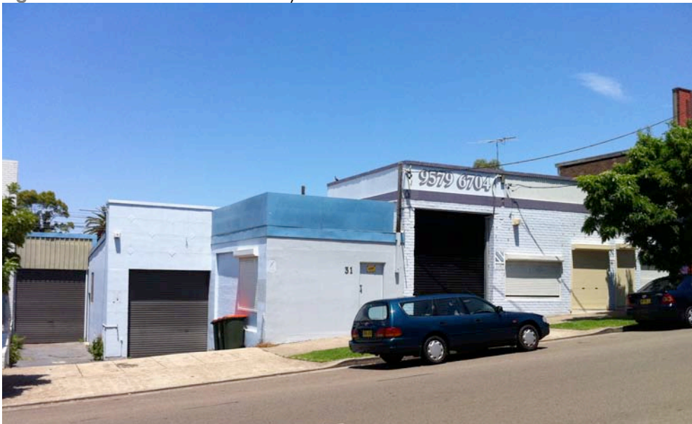
Figure 12 - View of 31 - 33 Treacy Street
