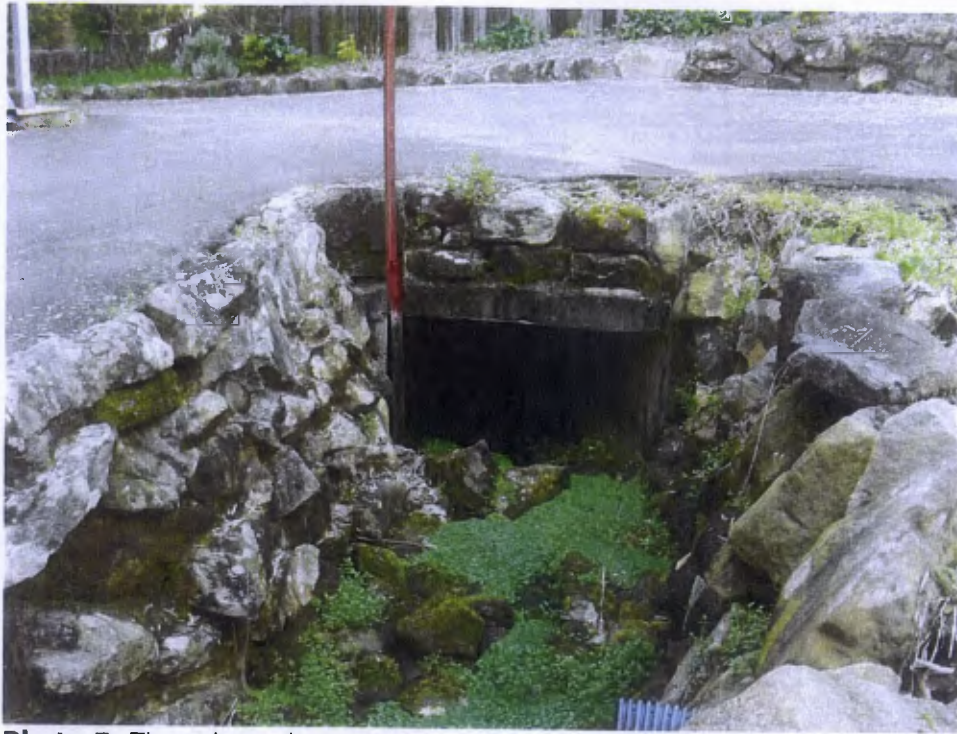
Photo 5: The culvert that conducts water collected from the 'riparian' drainage channel bisecting the site underneath the driveway to 1 Arilla Road and also underneath Arilla Road itself to the creek downstream located on the south-western side of Arilla Road.
