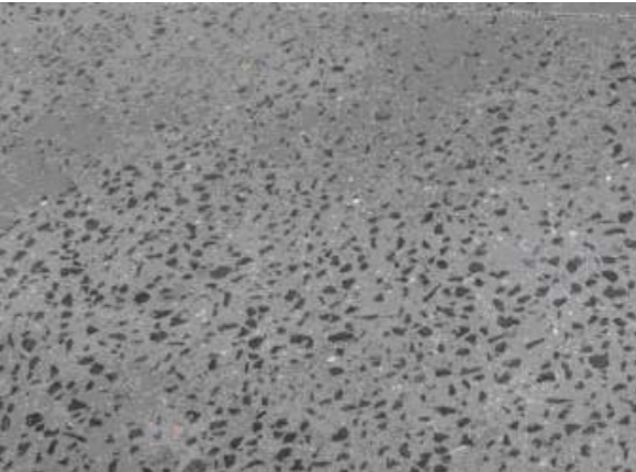
Insitu Concrete - Exposed Aggregate
