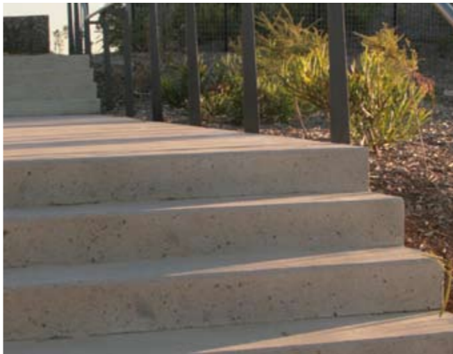
Concrete formwork stairs
