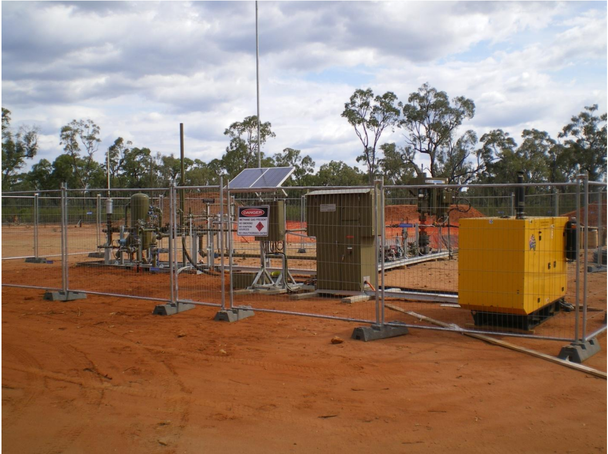
Plate 1: Example of vegetation clearing required for a typical well
