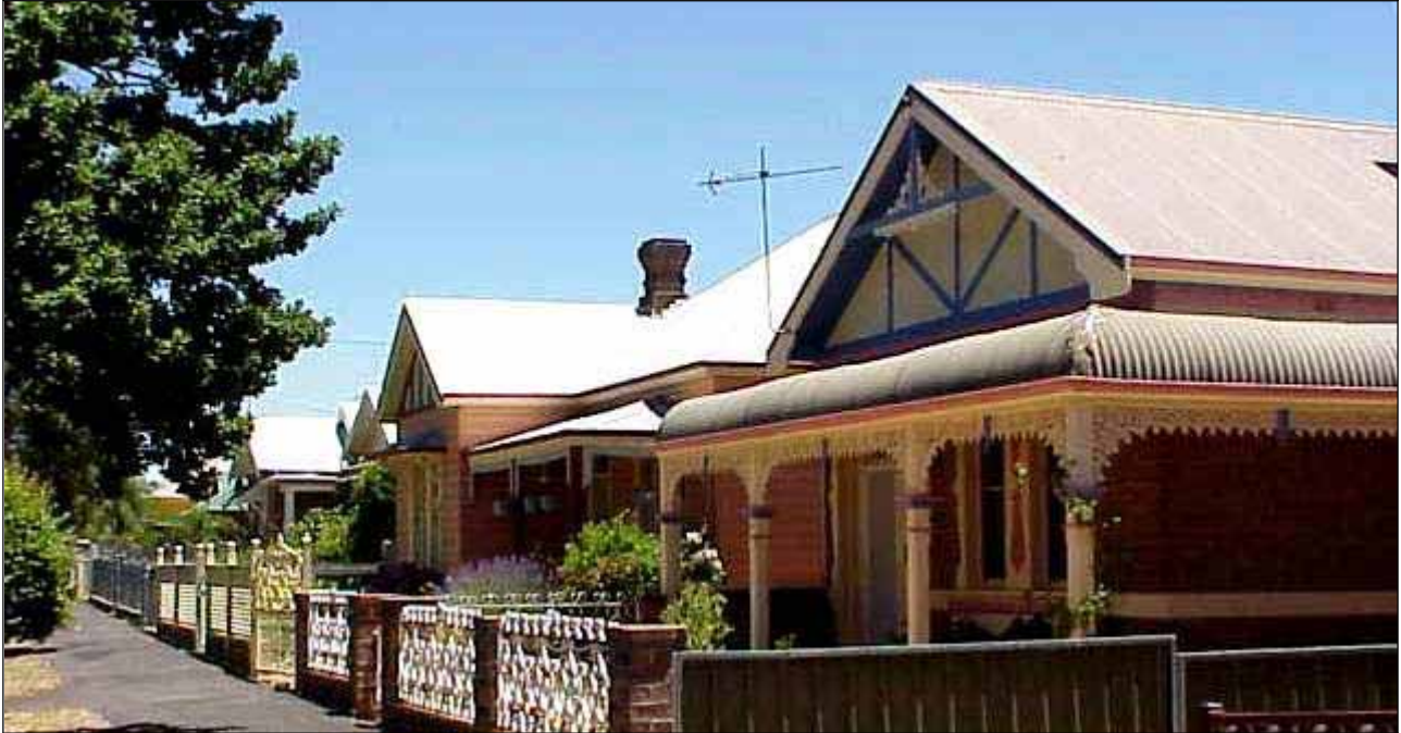
Photograph - Dora Street houses – Dora Street is a focus for the “village character” of East Orange
