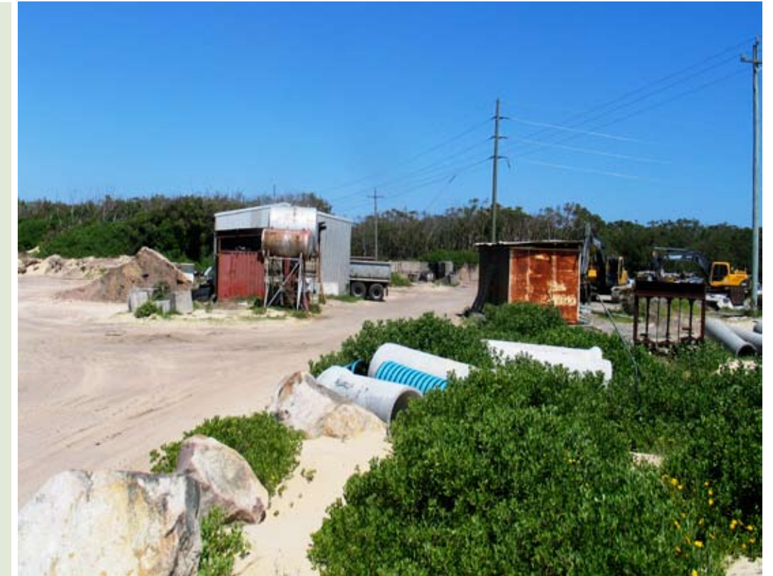
LOOKING TOWARDS EXISTING MACHINERY SHEDS ON THE SITE >
