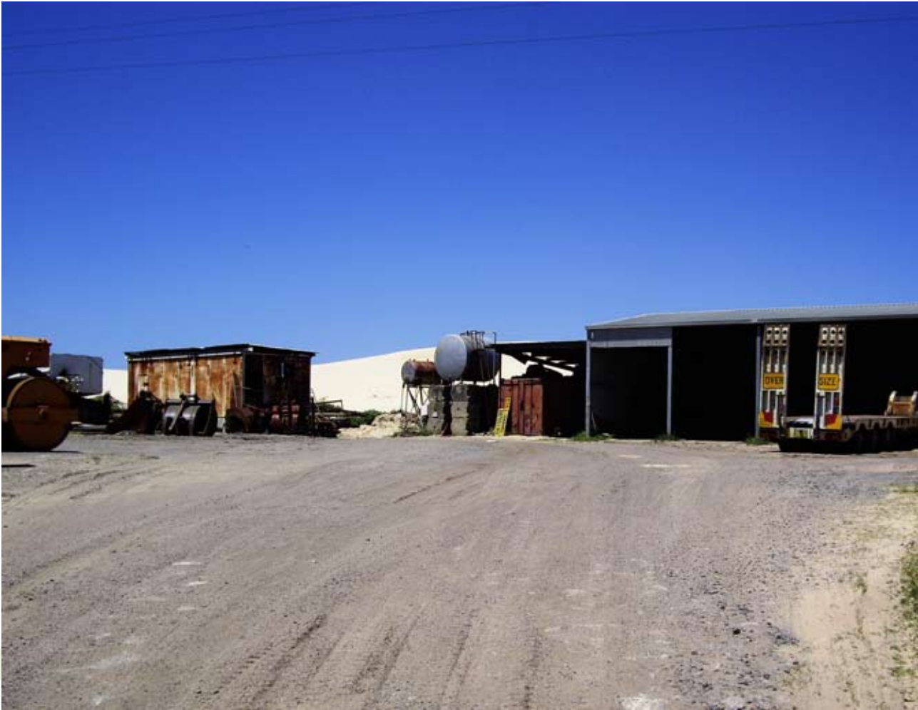
^ LOOKING SOUTH TOWARDS EXISTING SHEDS ON THE SITE
