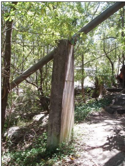
Figure 06 (below): Concrete pedestal and pipeline Source: Author, October 2007
