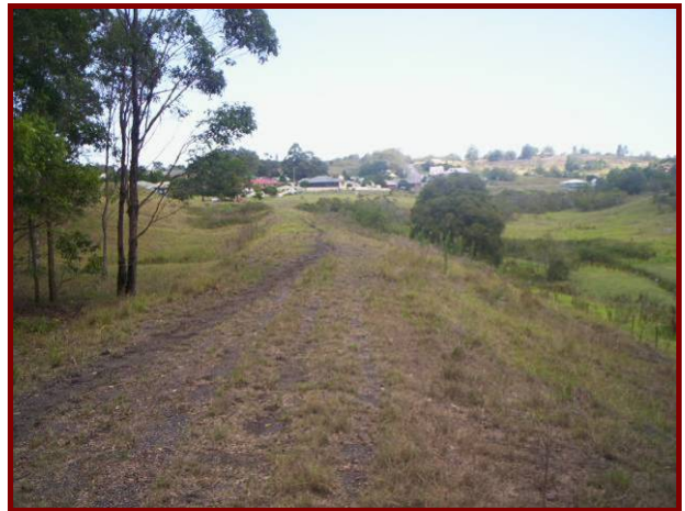
Photo 11 – Fill embankment from former rail line
