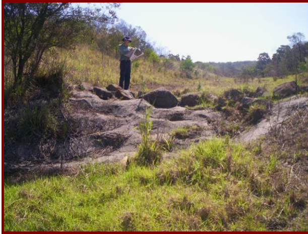
Photo 14 – Drainage structure in former open cut
