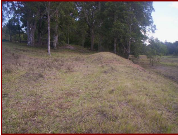
Photo 8 – Filled batter on western side of former railway, to the east of the open cut screens
