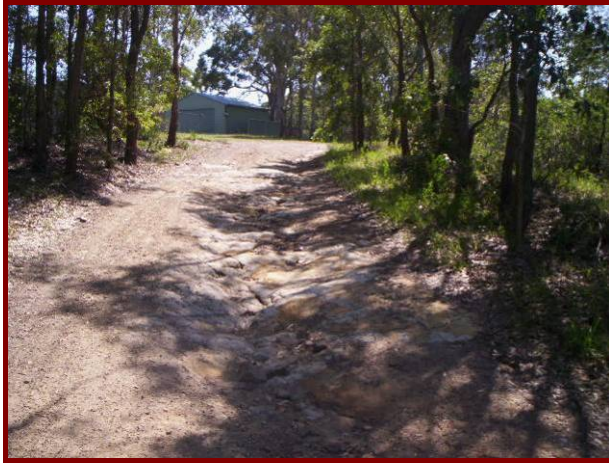
Photo 28 – Rock exposed at northern end of access track
