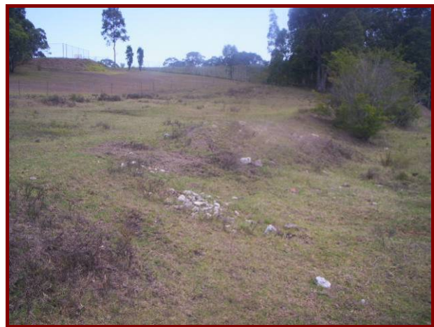
Photo 7 – Mounded filling including building rubble
