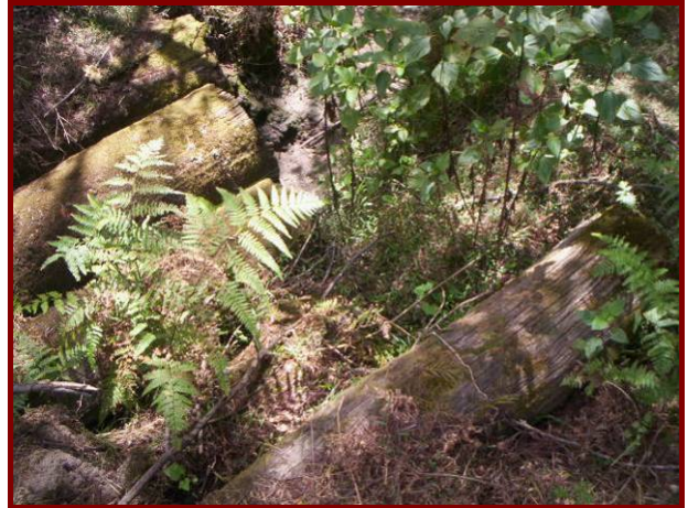
Photo 65 – Remnant Timber Bridge
