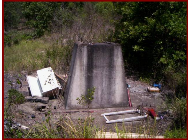
Photo 70 – Concrete Footing next to capped shaft
