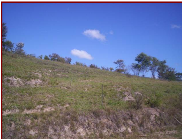
Photo 53 and 54 – Disturbed and slumping slopes near former Browns Colliery
