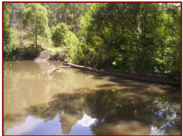
Photo 67 – Masonry Walled Dam
