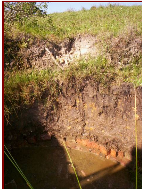
Brick Cistern at Reported Location of Pothole P6
