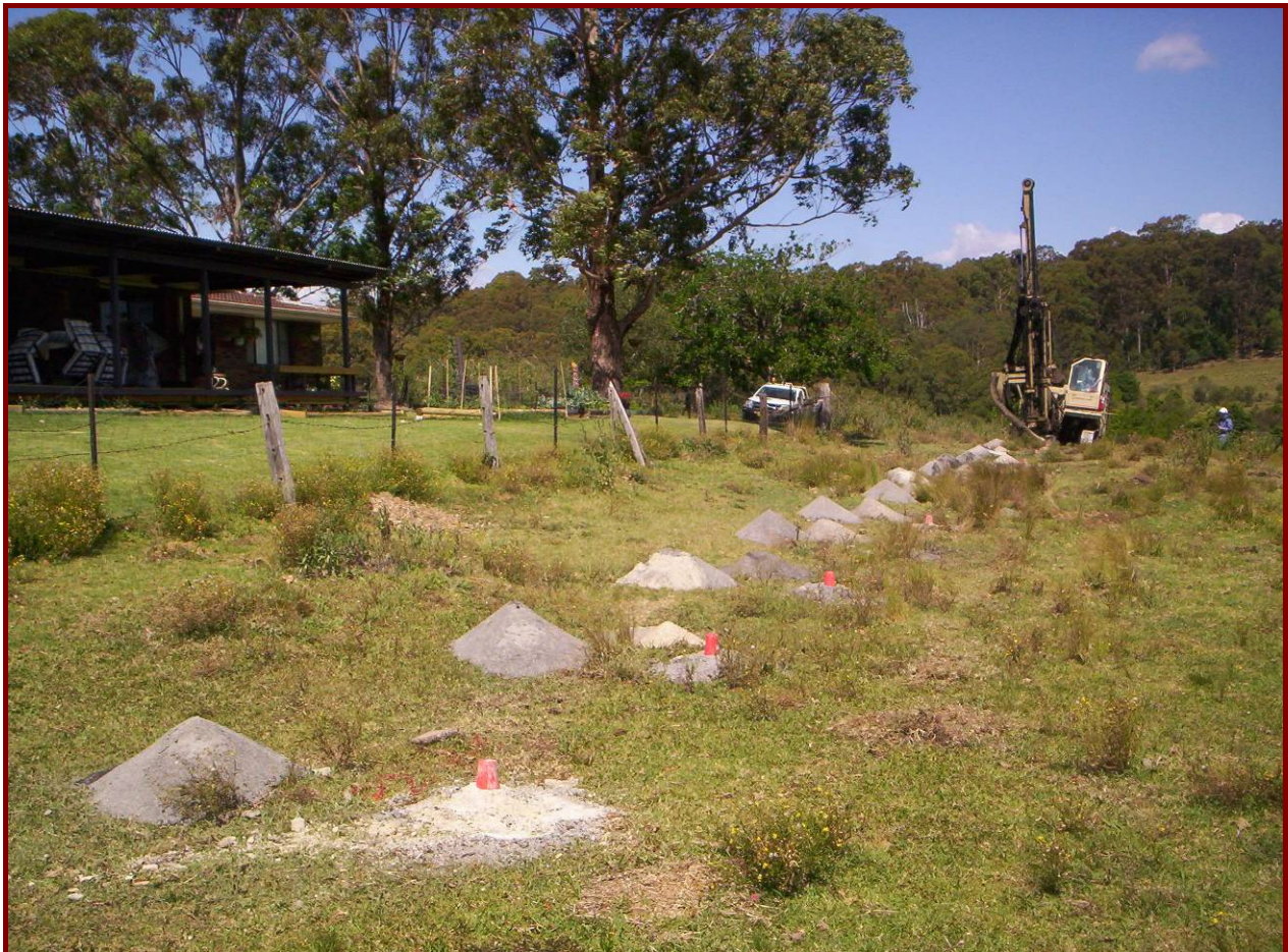
Percussion Drilling in Minmi West
