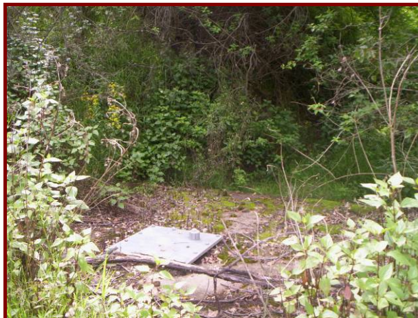
Capping on Shaft No 12
