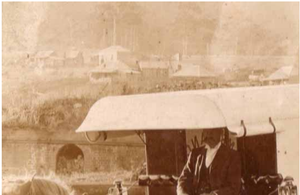
Photograph E.2 Source: Minmi Historical Society. Crop of a Minmi Ambulance Station photograph, facing southwest (date unknown). Coincidentally it shows a faction of the Minmi Coke Ovens.
