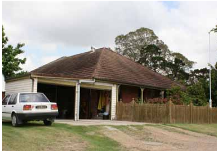
Photograph 5.1 Former Minmi Reservoir Residence. View from north east (ERM 2007) Former Minmi Public School, 196 Woodford Street
