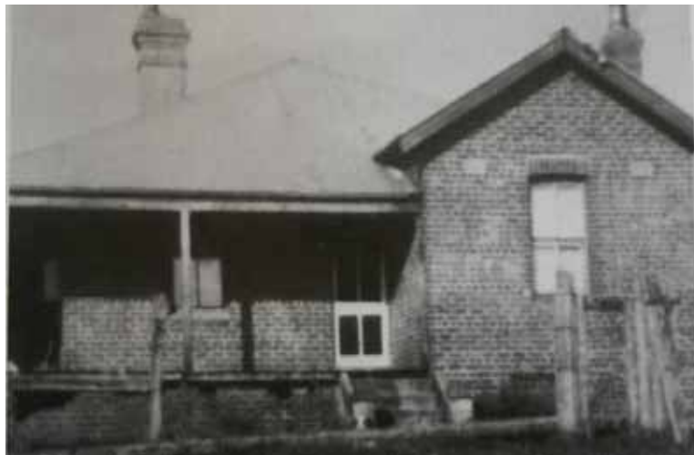
Photograph 5.23 John Brown's model Farm which has since been demolished (from personal collection of Kerry Hinds)
