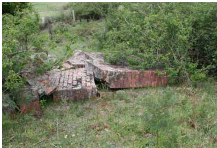
Photograph 5.22 View of collapse tank stand piers (ERM 2007)
