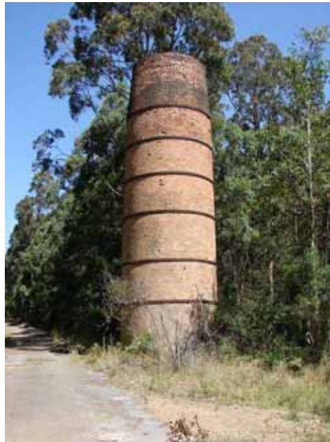
Photograph 5.25 Air Furnace Shaft Duckenfield No 2 (ERM 2007)
