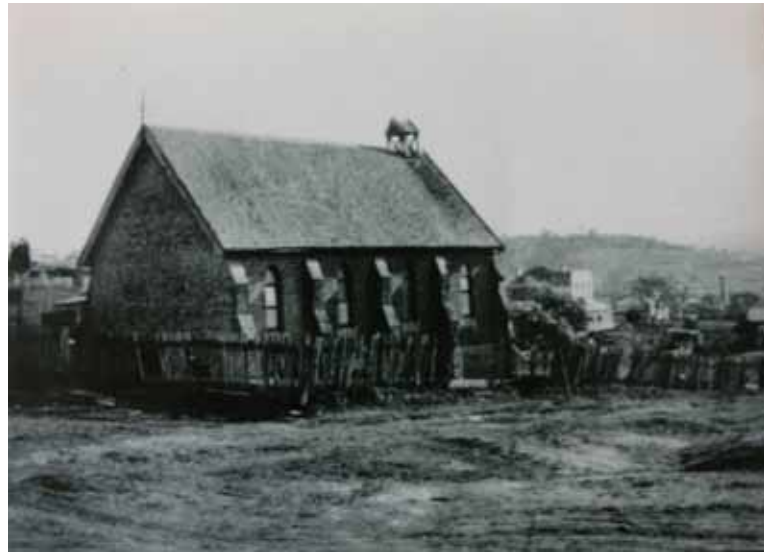
Photograph 5.37 View from the north east (from personal collection of Kerry Hinds).
