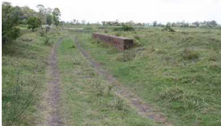
Photograph 5.21 Railway Siding viewed from south (ERM 2007)
