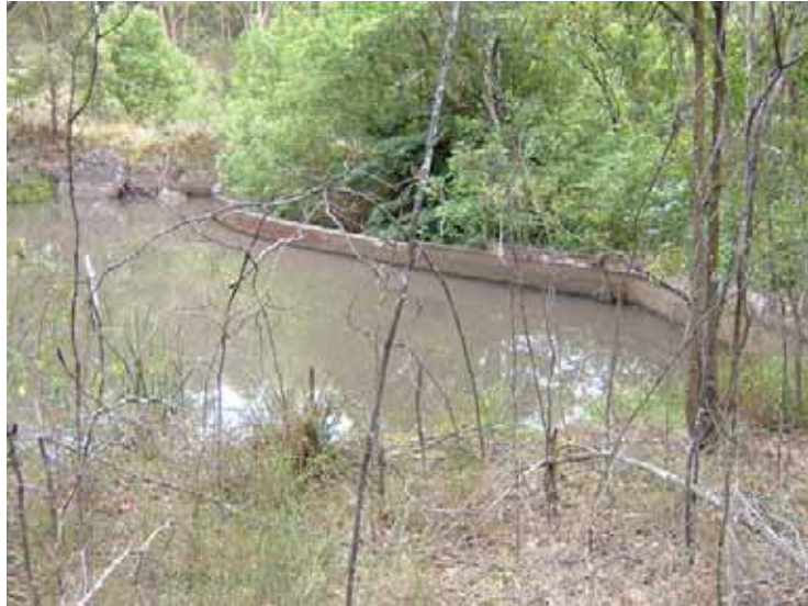
Photograph 5.40 Wall of the brick dam
