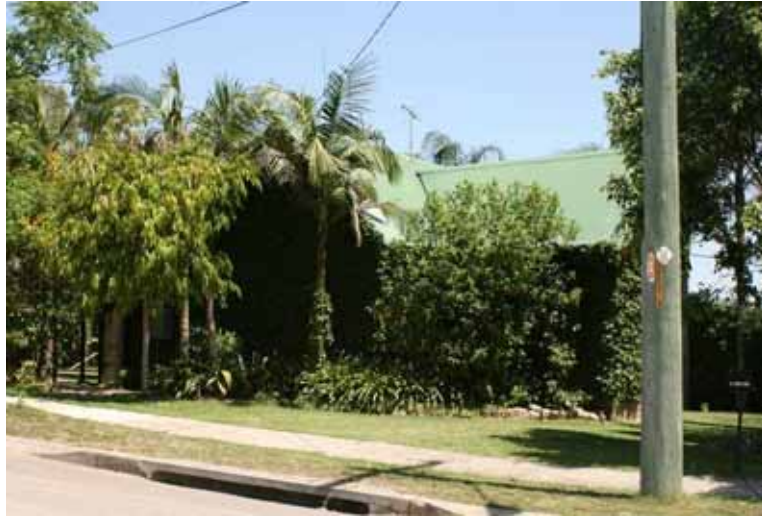
Photograph 5.39: Former Church Manse from north east.
