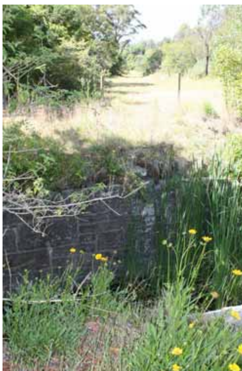
Photograph 5.6 View south east over Minmi Creek showing bridge abutments and railway alignment along the valley floor (ERM 2007)
