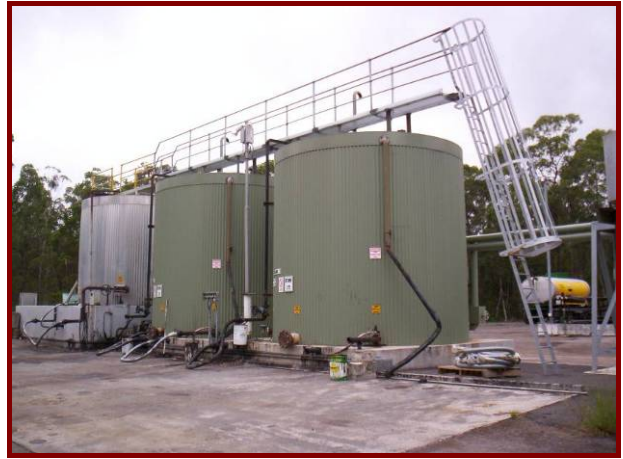
Photo 16 – Aboveground bitumen and kerosene coated storage
