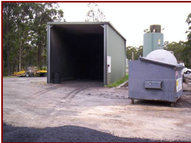
Photo 11 – Spray seal vehicle washdown bay (kerosene used)
