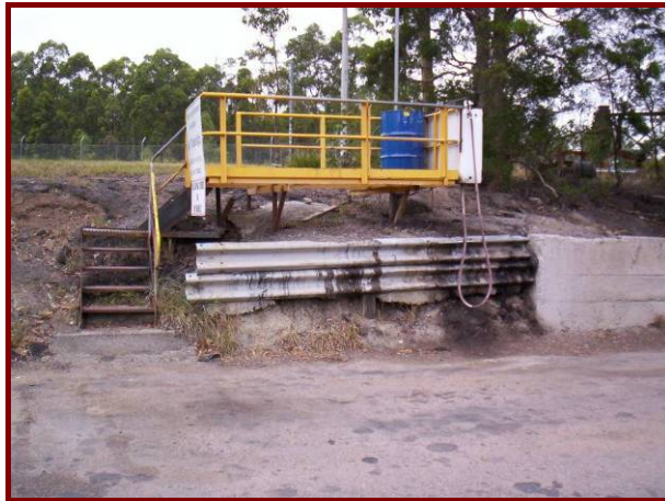
Photo 6 – Surface hydrocarbon staining adjacent to the asphalt plant area
