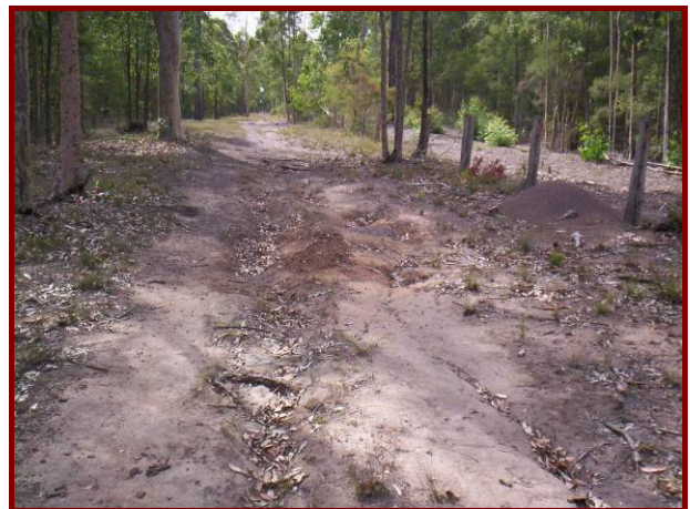
Photo 31 – Local erosion on the access track on the southern site boundary
