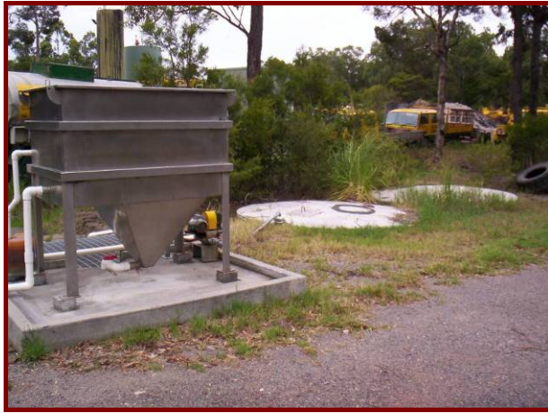
Photo 15 – Oil water separator (runoff from diesel aggregate stockpile area)
