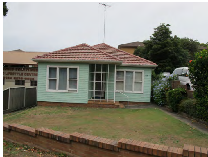
538 RAILWAY PDE VIEW FROM RAILWAY PDE
