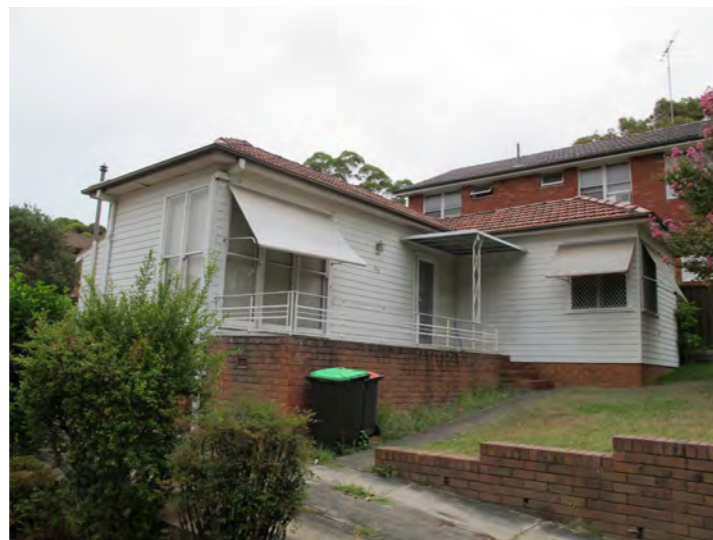
540 RAILWAY PDE VIEW FROM RAILWAY PDE
