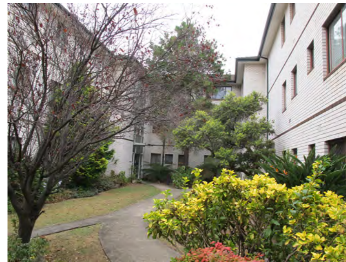
10-14 ST GEORGES PDE VIEW INTO COURTYARD
