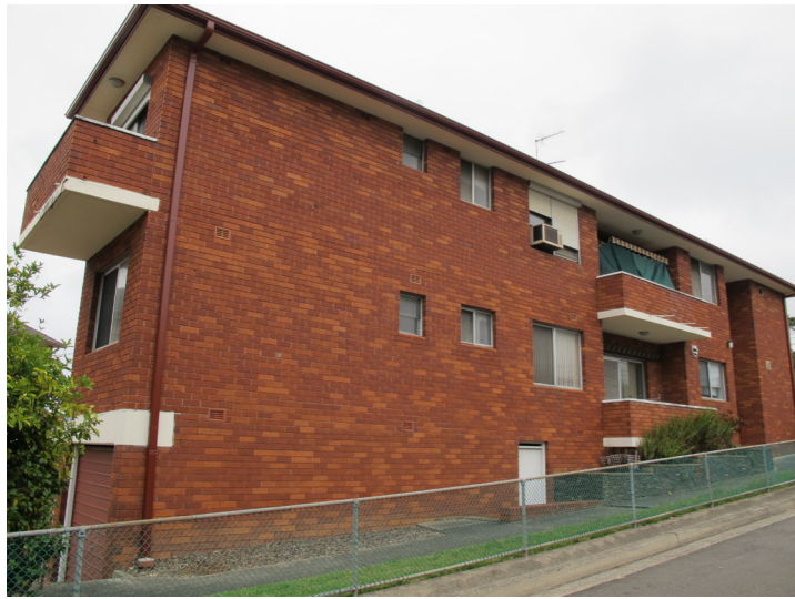
552 RAILWAY PDE VIEW FROM COW LANE 3ST(2R)
