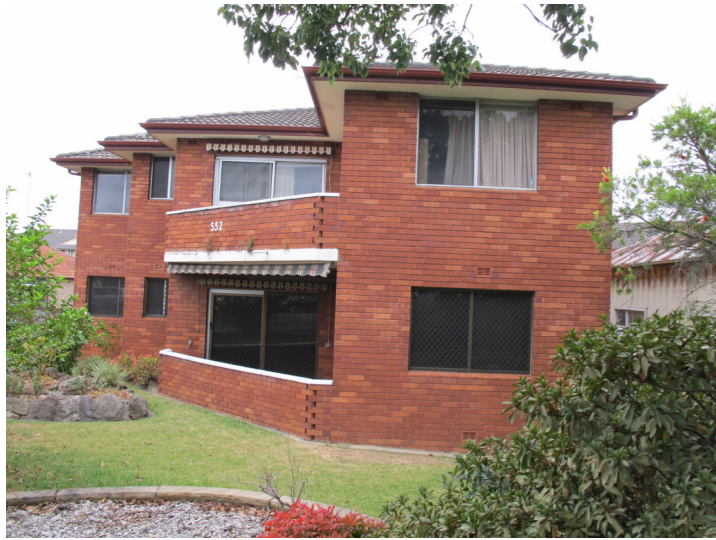
552 RAILWAY PDE VIEW FROM RAILWAY PDE 3ST(2R)
