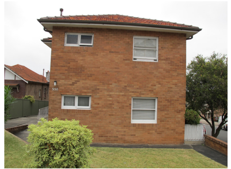
558 RAILWAY PDE VIEW FROM RAILWAY PDE 3ST(2R)
