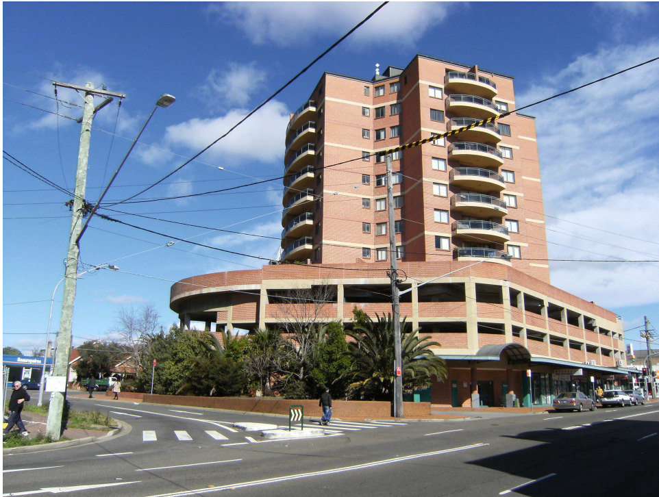
Figure 5: High rise development at the corner of Treacy Street and The Avenue
