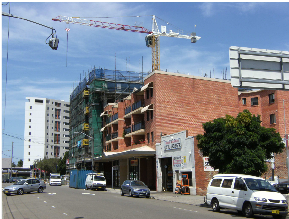
Figure 4: Development to the east of the site
