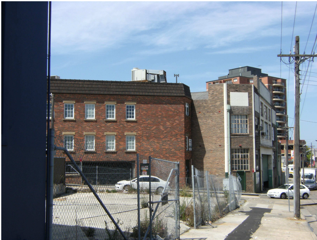
Figure 3: Existing development along Treacy Street to the north of the site
