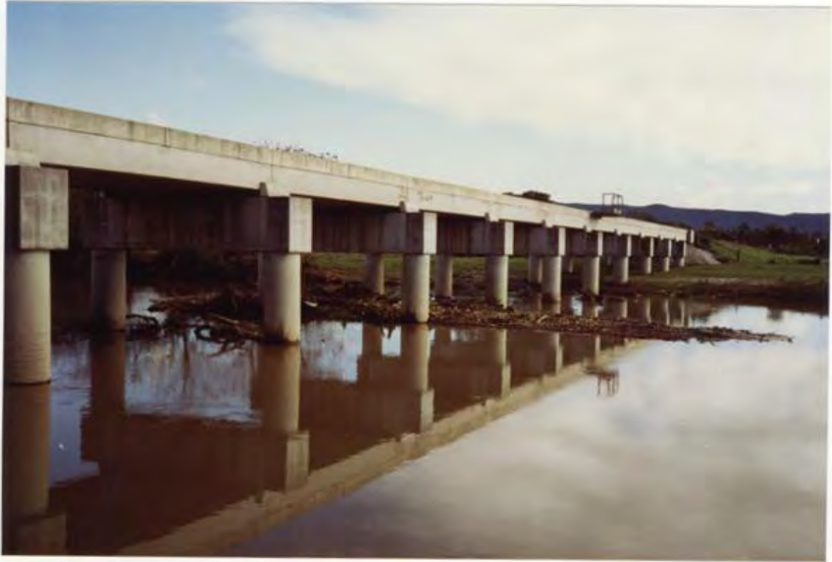
Rail Bridge - Accumulated Debris After Event From DS South Bank
