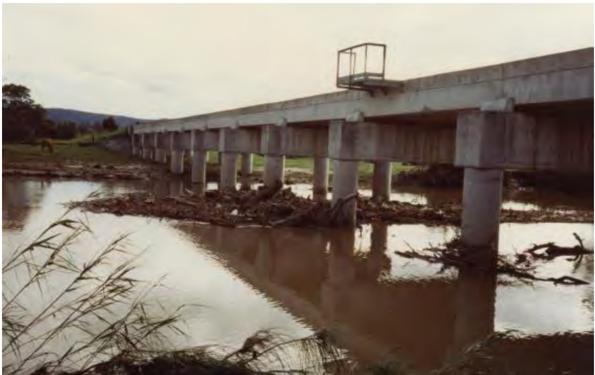
Rail Bridge - Accumulated Debris After Event From US South Bank
