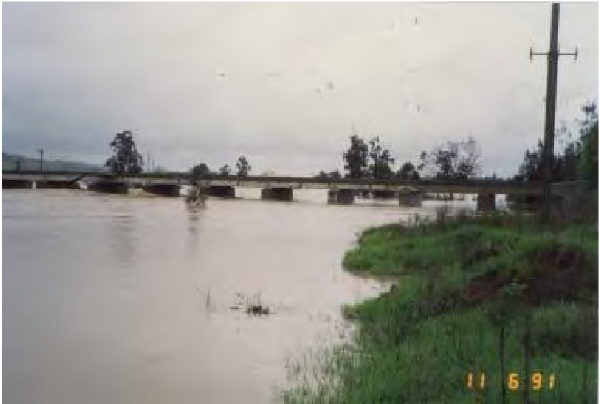
1..US RAIL BRIDGE (Note afflux above central spans)
