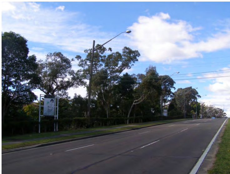
Figure 6 – The south-western boundary of the site, viewed from the west on Epping Road
