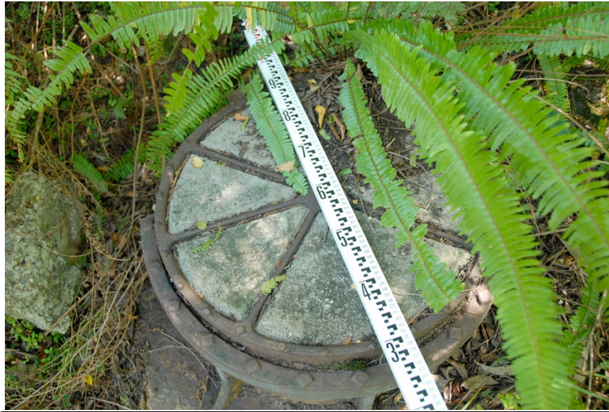
Plate 7: Manhole cover for sewer pipe located on the walking track
