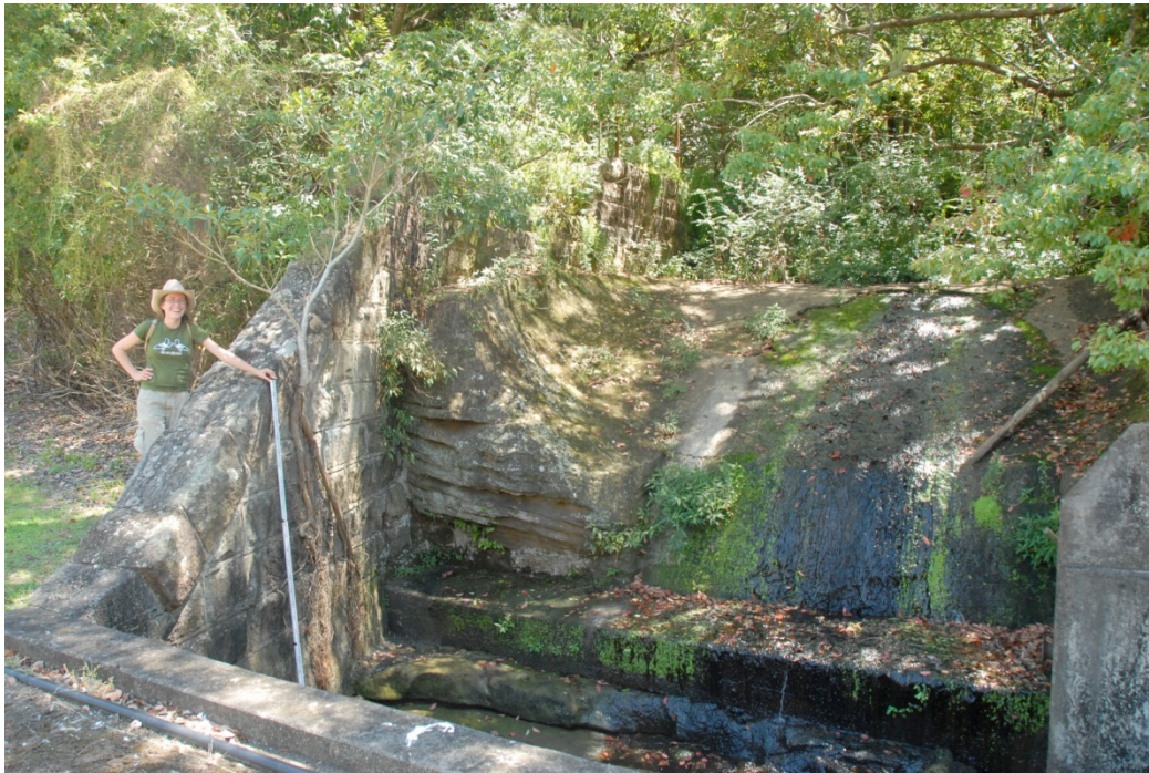
Plate 5: Sandstone walls just downstream from the weir, facing north
