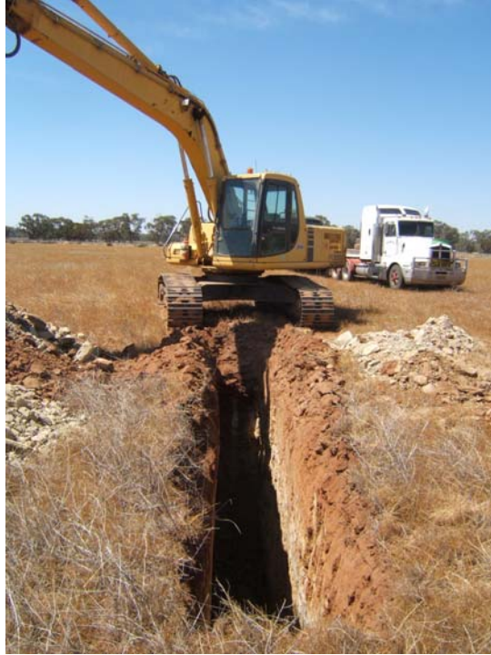
Excavator and typical test pit
