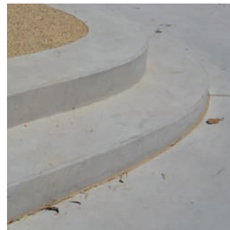
Cove Finish Stairs
