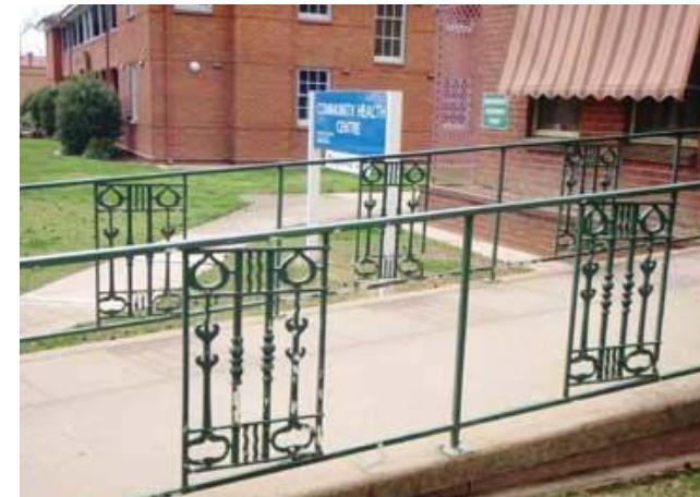
Recycled Balustrade from Old Hospital Building
