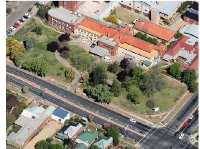
Landscaping to the north of site prior to tree removal in accordance with the Arborist Report
