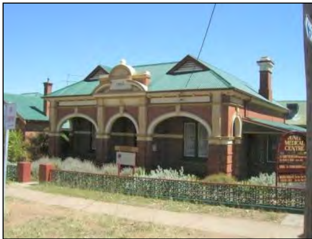
Figure 13: Medical Centre (former School of Arts), Junee State Heritage Inventory, Database No. 1840154.
