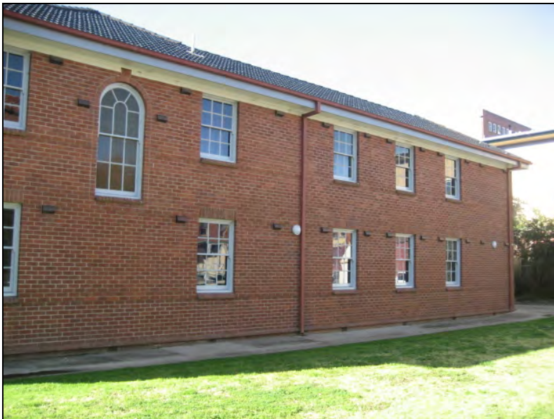
Figure 150: Southern elevation, detail.
