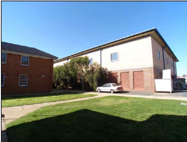
Figure 144: Side and rear of the Clinical Services Building.
