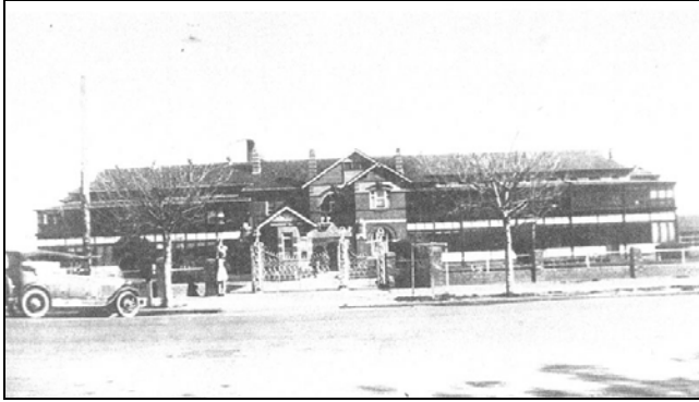
Figure 31: New boundary wall to the front of the Hospital.
