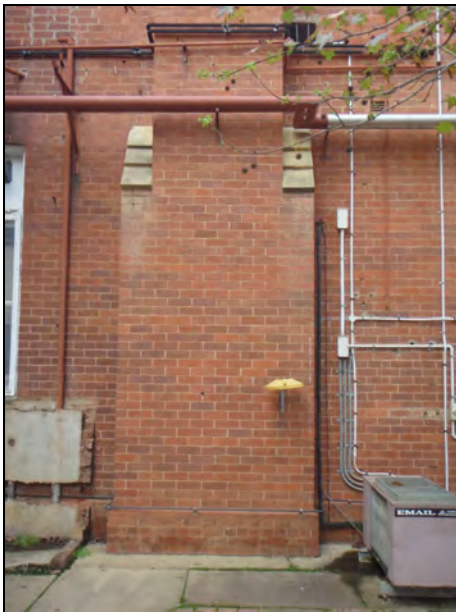
Figure 94: Detail of an original chimneybreast, rear of 1922 wing.
