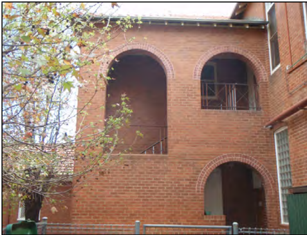
Figure 92: Staircase, 1922 wing, showing detailed brick arches and wrought iron balustrades. Note also later glass blocks filling in an original window opening. The first floor windows above are original.
