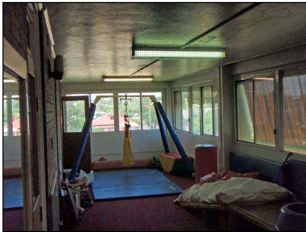
Figure 141: Within the enclosed verandah. The original windows have been replaced.
