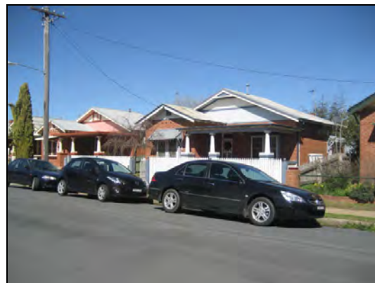
Figure 166: Nos. 14 and 16 Yabtree Street.
