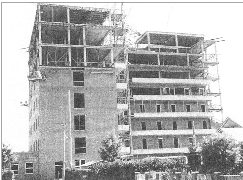
Figure 37: The Multi-Storey Block under construction.
