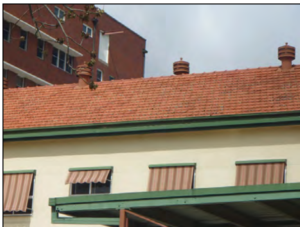
Figure 87: Detail of the original roof vents on the 1910 building.
