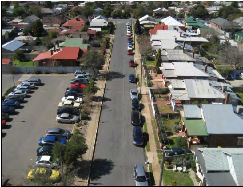
Figure 68: Yabtree Street, looking west, from the roof of the upper levels of the Main Building.
