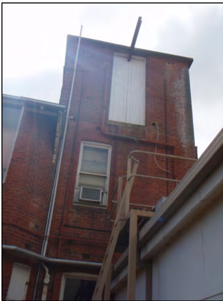
Figure 90: Remnants of the hoist, southern elevation.
