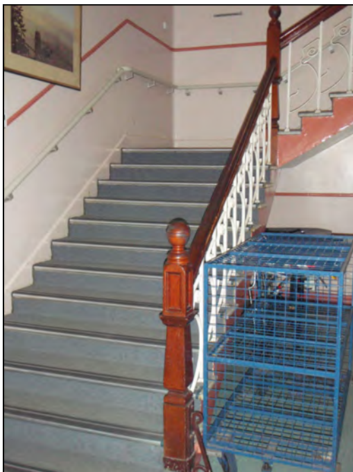
Figure 102: Detail of the original stair balustrade.
