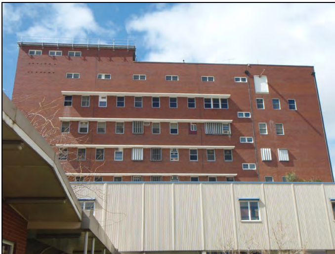
Figure 113: The western elevation.
