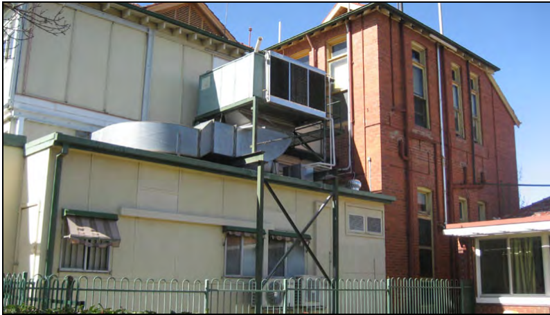
Figure 89: The western elevation of the 1922 wing.
