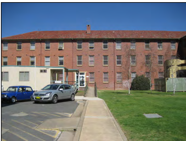
Figure 138: Southern elevation of Lewis House.
