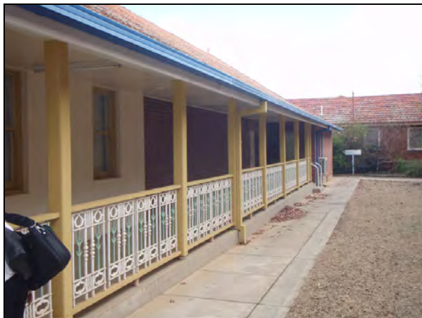
Figure 158: Physiotherapy Block, showing detail of the re-use of the Old Hospital balustrade.
