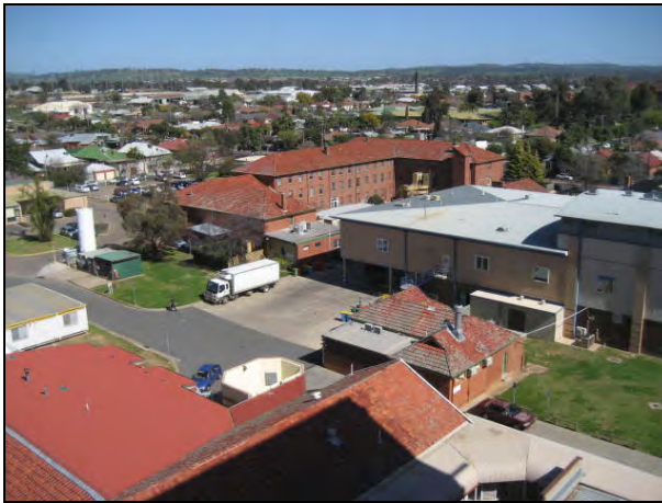
Figure 137: View to the rear of Lewis House from the roof of the Main Hospital Building.
