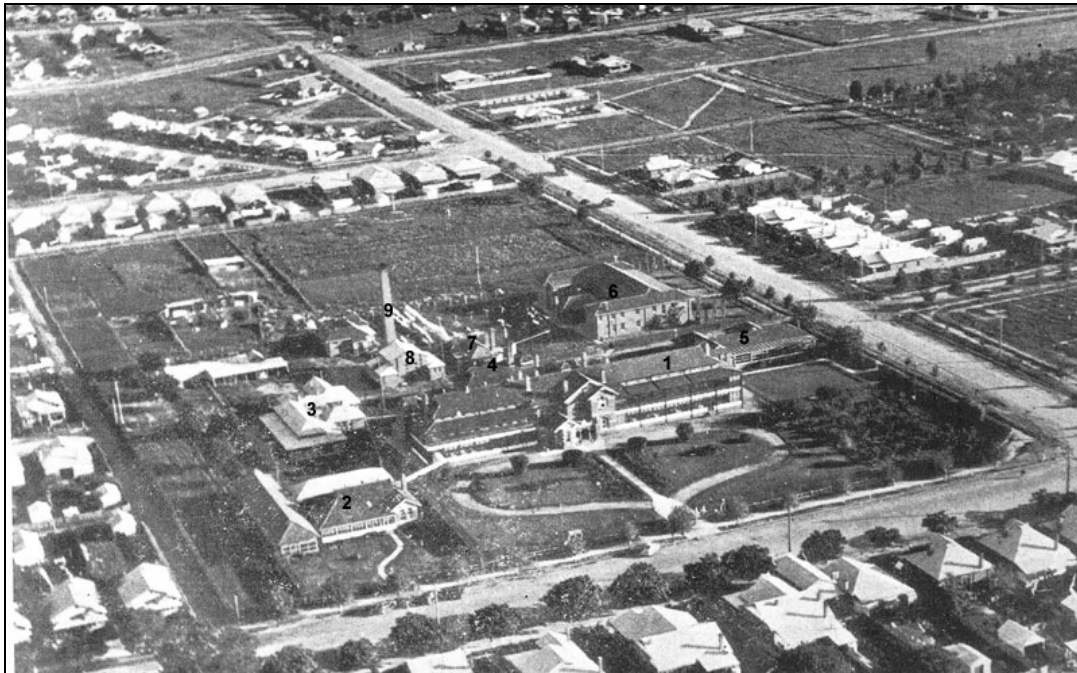
Figure 32: Aerial photograph of Wagga Wagga Hospital, 1943.
