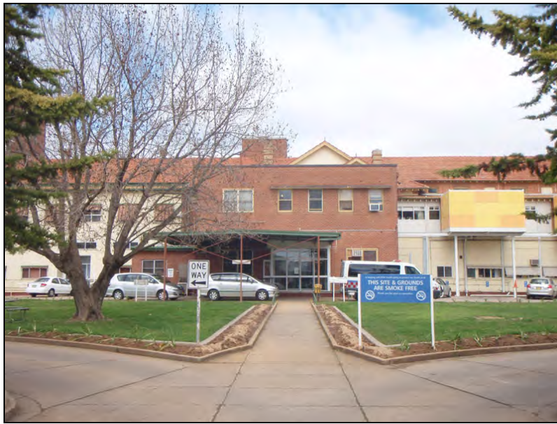
Figure 82: Northern elevation of the 1944 Administration Block, above which can be seen the gables of Vernon's original entrance and two banded brick chimneys.
