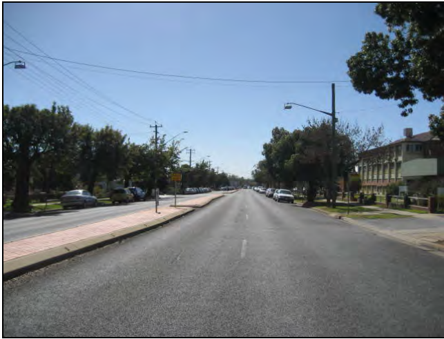
Figure 58: Docker Street, looking east. Lewis House is visible on the right hand side.
