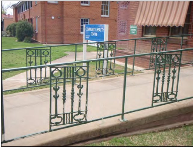
Figure 95: Recycled balustrade from the 1909 building re-used as a handrail outside the Community Health Centre.
