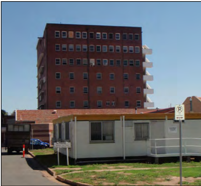
Figure 112: The southern elevation.
