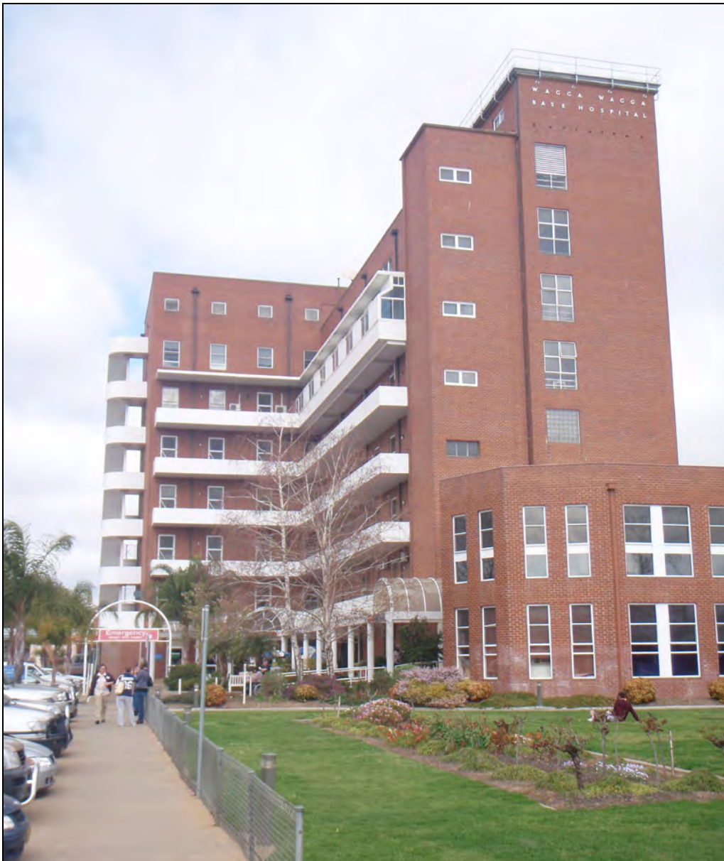
Figure 104: Looking south towards the Main Building. The two storey section on the northern side, the fire stair and the ground floor colonnade are later additions to the original building.
