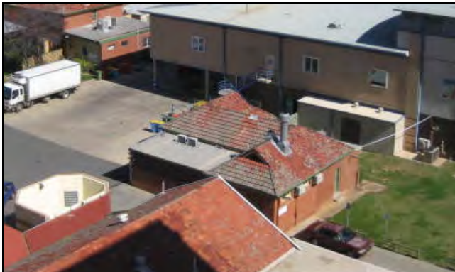
Figure 118: Looking down over the mortuary.
