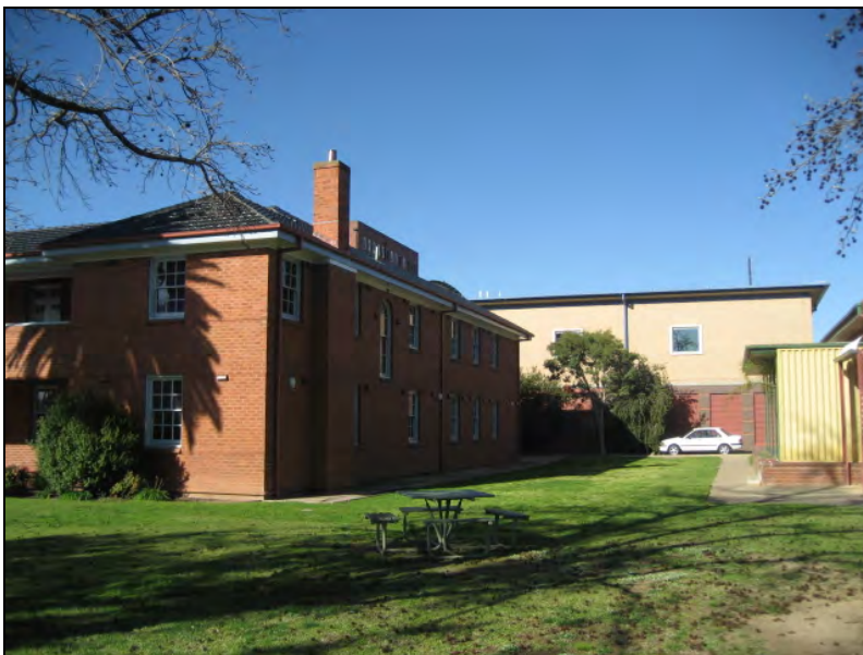
Figure 148: The southern elevation.
