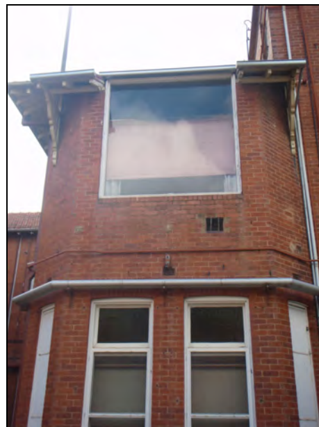
Figure 91: Bay containing the original Operating Theatre, showing window and decorative timber brackets.
