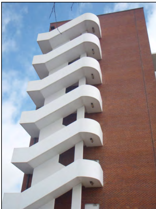
Figure 111: Detail of the Fire Stair built in 1986. This stair has strong echoes of Wells Coates' iconic staircase at the Isokon Flats, Hampstead (1933-4).
