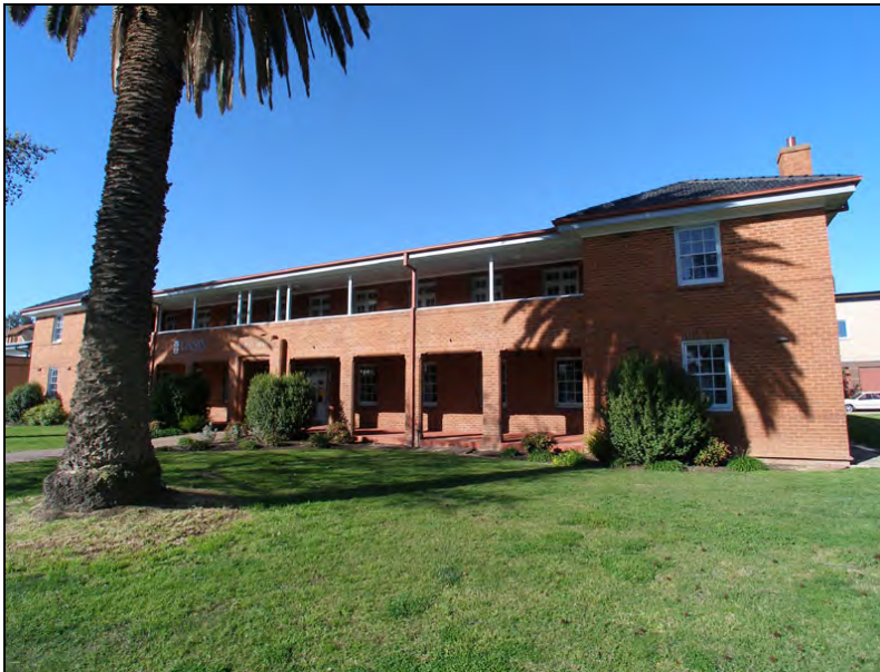
Figure 146: The eastern elevation
