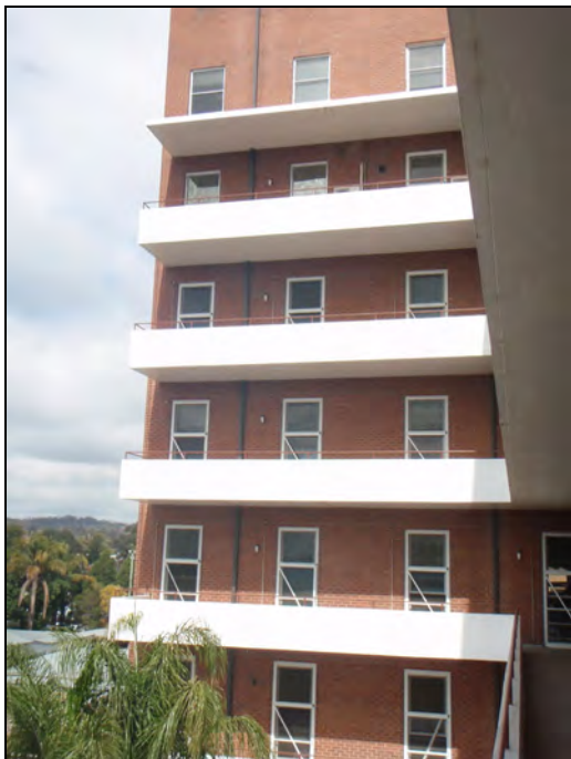
Figure 108: Detail of the eastern elevation, showing the regular pattern of triple hung windows and screen doors.
