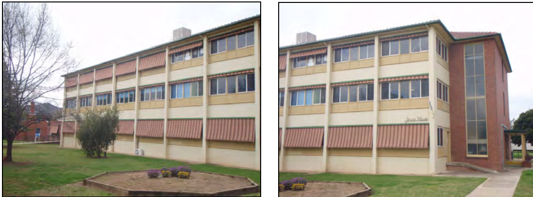
Figure 132: Docker (eastern) Street elevation of Lewis House, southern end. Note the stylised 1960s-style wrought iron lettering 'Lewis House.'
