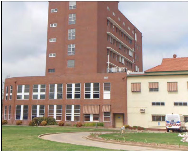
Figure 80: Northern elevation of the later brick addition at the western end of the building.
