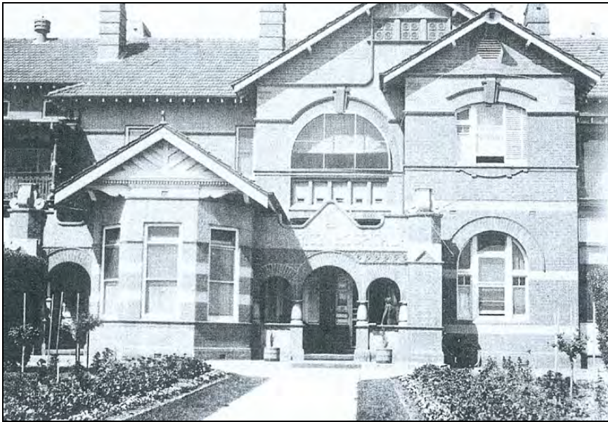
Figure 22: An undated photograph of the front entrance, showing the original, fine detailed brickwork contrasted with sections of roughcast render. Note also the carefully planted garden beds.
