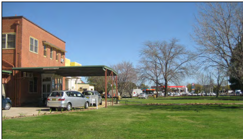
Figure 83: The port-cochere, a later addition to the 1946 Administration Block
