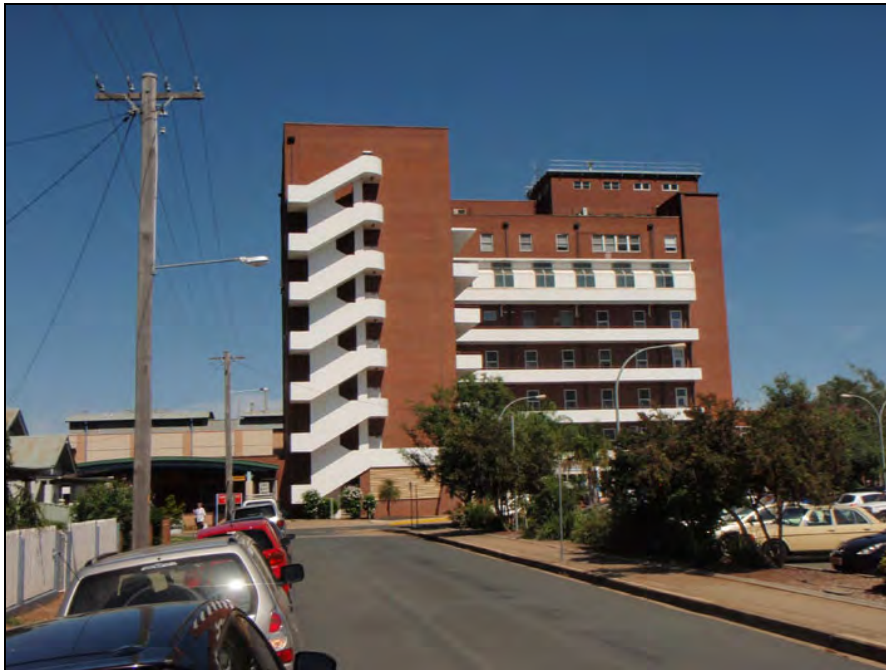
Figure 110: Looking west towards the Main Hospital Building showing the fire stair on the eastern elevation of the east-west running section of the building and the east facing balconies of the north-south section of the building.
