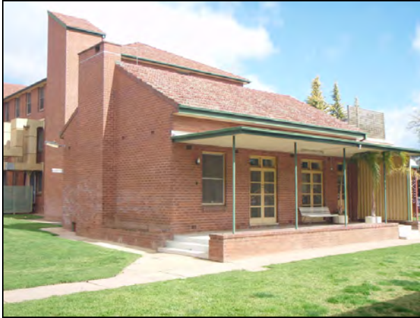
Figure 136: Behind the Community Services wing. These doors have original timber flyscreens.
