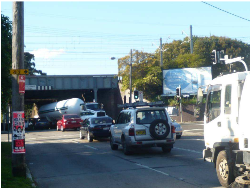
View looking north along Old Canterbury Road at Railway Terrace. Old Canterbury Road is one lane northbound under the overpass.
