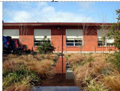
Linear bioretention system to treat runoff from southern part of site, including blocks A, E and F
