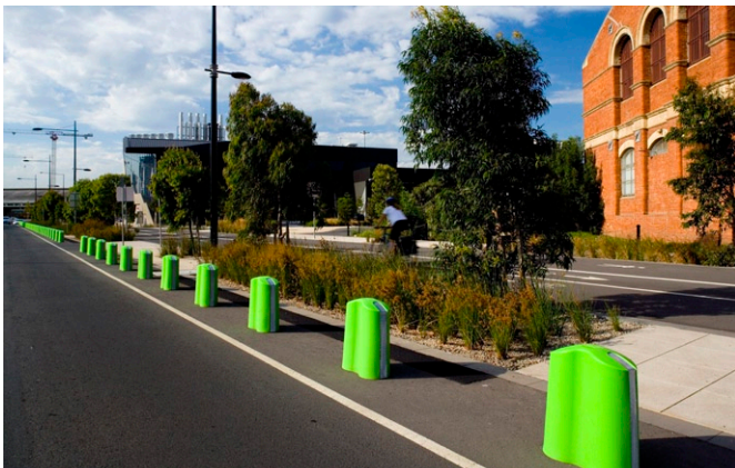
Stormwater bioretention within road reserve
