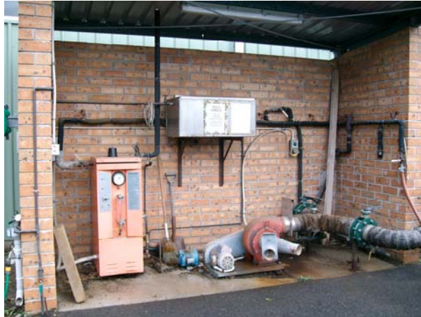
Photo 3 – Electric sterilising unit with minor staining on the concrete base.
