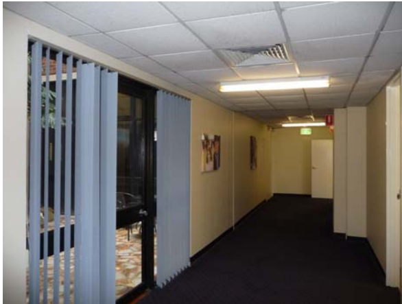
Typical hallway, offices and courtyard, ground floor
