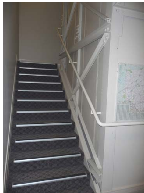
Stair and enclosed lift well
