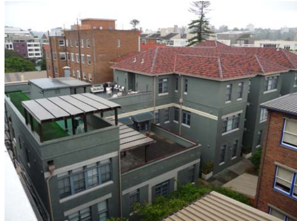
Roof and rear extension
