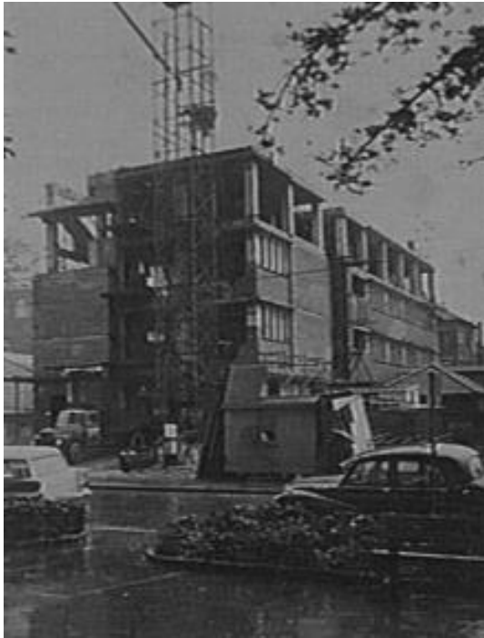
Figure 23 – Construction of the Moncrieff Barron Wing, 1964
