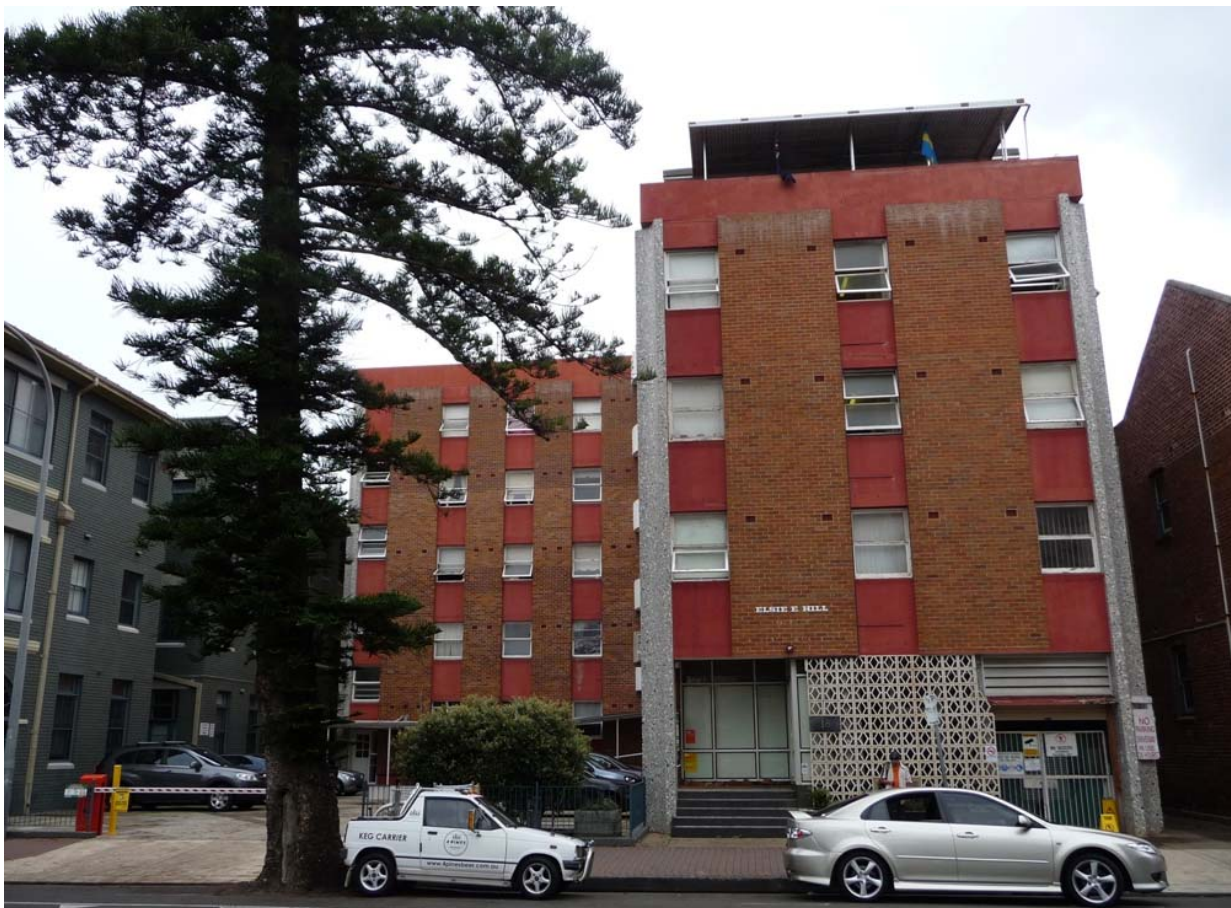
Figure 9 – Elsie Hill building
