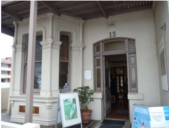
Ground floor, south section and main entry
