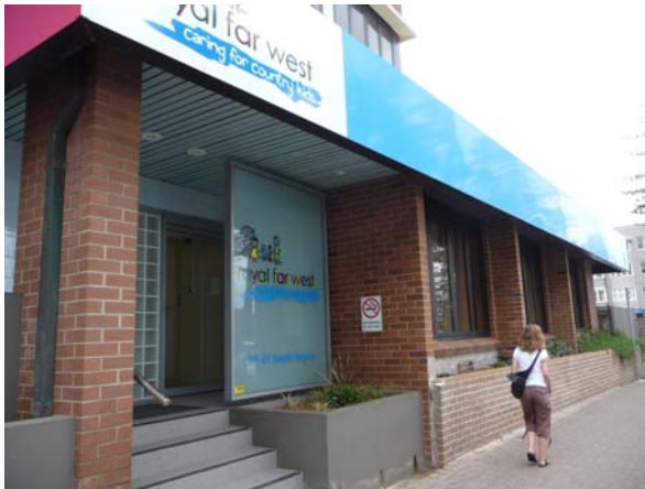
Detail of main elevation ground floor
