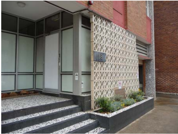
Main entry from Wentworth St
